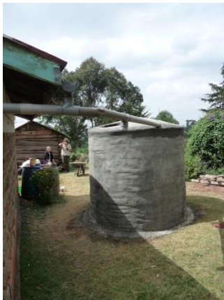
Fig's 7 and 8: Completed tank and filling.
