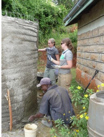
Fig's 5 and 6: Plastering the outside wall, constructing the domed roof.
