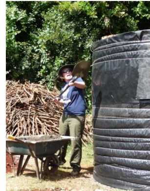
Fig's 2, 3, 4: Foundation wire, wall frame, plastic wrapped walls with plaster being shoveled in by student.
