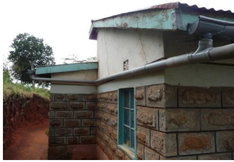
Fig 1: Gutter system on main house.
