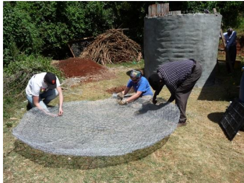
Fig's 5 and 6: Plastering the outside wall, constructing the domed roof.
