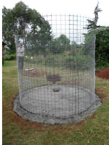
Fig's 2, 3, 4: Foundation wire, wall frame, plastic wrapped walls with plaster being shoveled in by student.
