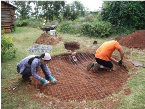
Fig's 2, 3, 4: Foundation wire, wall frame, plastic wrapped walls with plaster being shoveled in by student.
