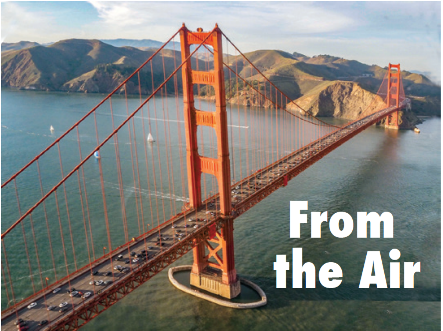
Golden Gate Bridge
