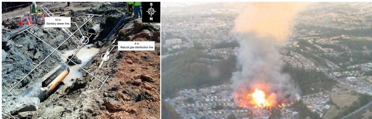
Figure 3: The 2010 San Bruno Gas Pipeline Explosion, Caused by System Pressure Changes, Killed 8 People
