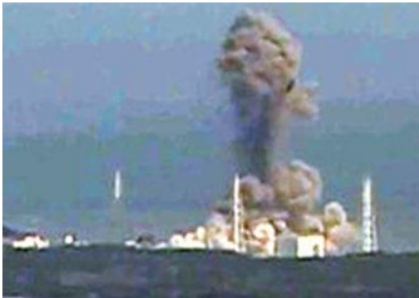
Figure 16: The Fukushima Explosion, 2011 (NEA)
