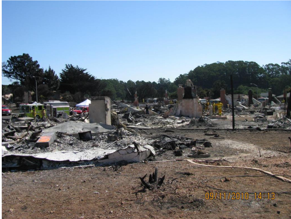
Figure 19: San Bruno Gas Pipeline Fire Damages that Killed 8 People
