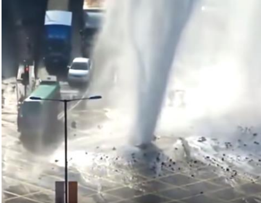
Figure 1: A Water Main Break Caused by Repeated Water Hammers ( https://www.youtube.com/watch?v=vp2G6hqRh1Q )
