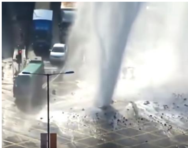
Figure 21: Pipeline Ruptured Due to Water Hammer
