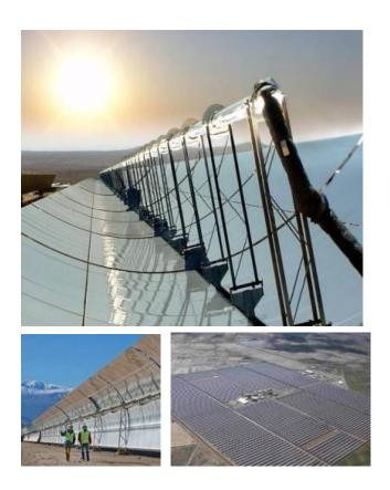
The parabolic troughs are used to track the sun and concentrate sunlight on to the thermally efficient receiver tubes placed in the trough focal line. In these tubes, a thermal transfer fluid is circulated, such as synthetic thermal oil. This oil is then pumped through a series of heat exchangers to produce steam. The steam is converted to electrical energy in a conventional steam turbine generator.
