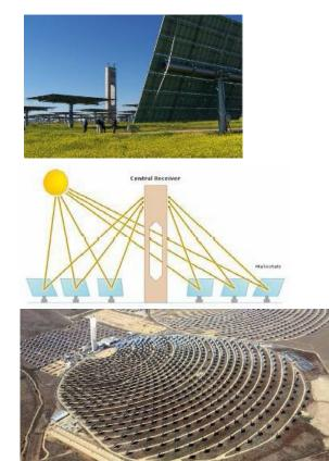
A circular array of heliostats (2 axis tracking mirror) is used to concentrate sunlight to a central receiver mounted on the top of a tower. A heat transfer medium in this receiver absorbs the highly concentrated radiation and coverts it into thermal energy to be used by a turbine.
