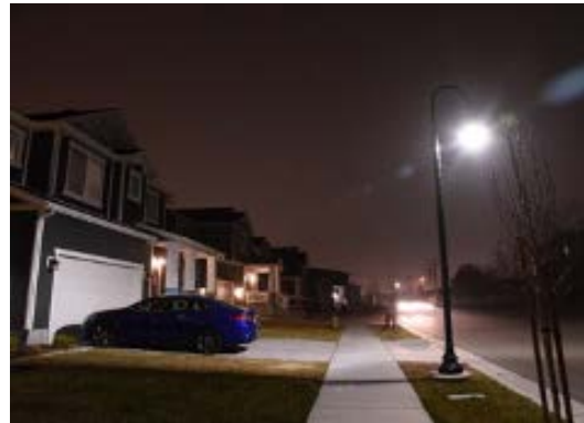
A pedestrian light with inappropriate light distribution and poor shielding creates a significant amount of light trespass on a nearby residence.
