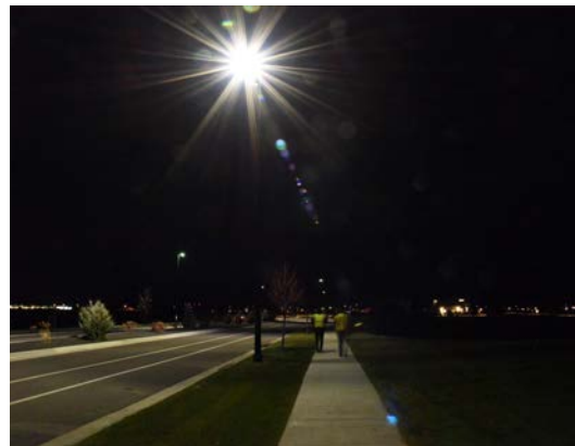
A well shielded street light with appropriate light distribution provides adequate light for the street and sidewalk with minimal light spill beyond the sidewalk.
