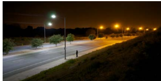
In the distance, the warm amber glow of low CCT (1800K) high pressure sodium street lights is shown in comparison to higher CCT (4000K) LED street lights in the foreground.
