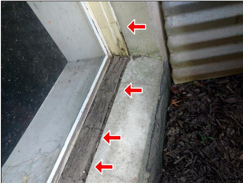
2.0 Item 14 (Picture) Basement window frame deteriorated
