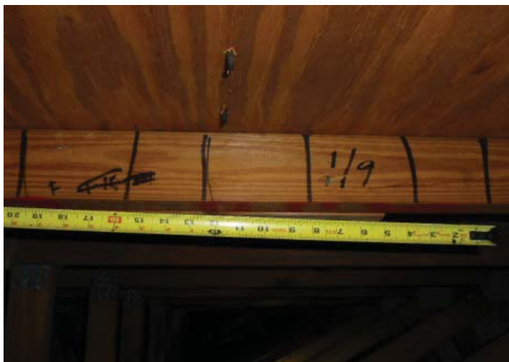
#3 ROOF DECK ATTACHMENT 6" X 6" NAIL SPACING
