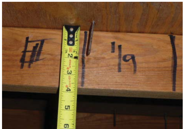
#3 ROOF DECK ATTACHMENT 8d NAILS
