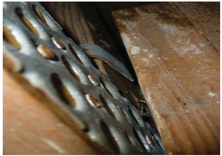
#4 ROOF TO WALL ATTACHMENT OPPOSITE SIDE
