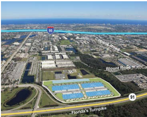
Rock Lake Business Center 3100 - 3250 NW 33rd Street Pompano Beach, Florida 494,425 SF for Lease
