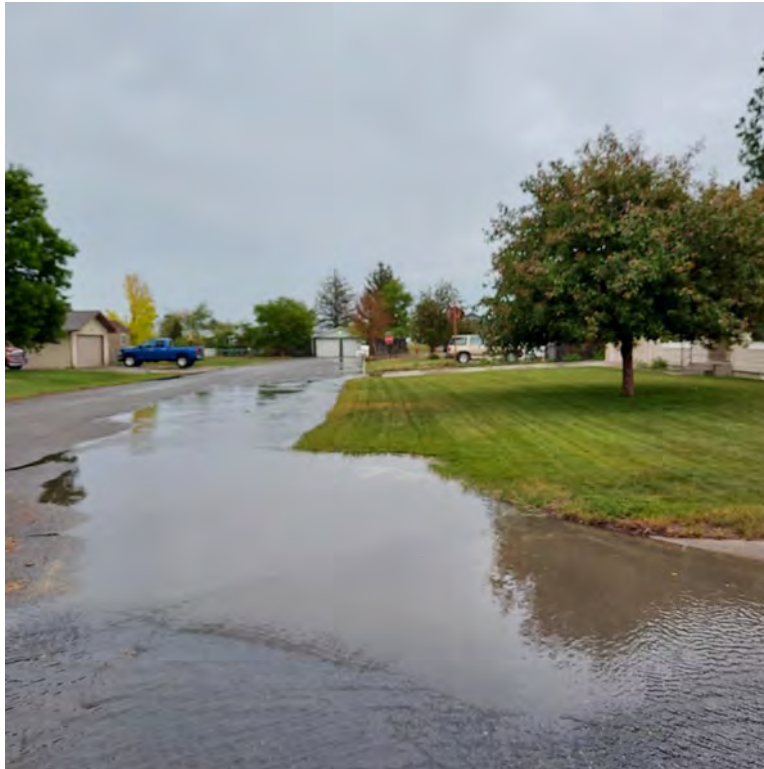
Photo 5: Flooding at Buffalo Road and Red Fox Drive
