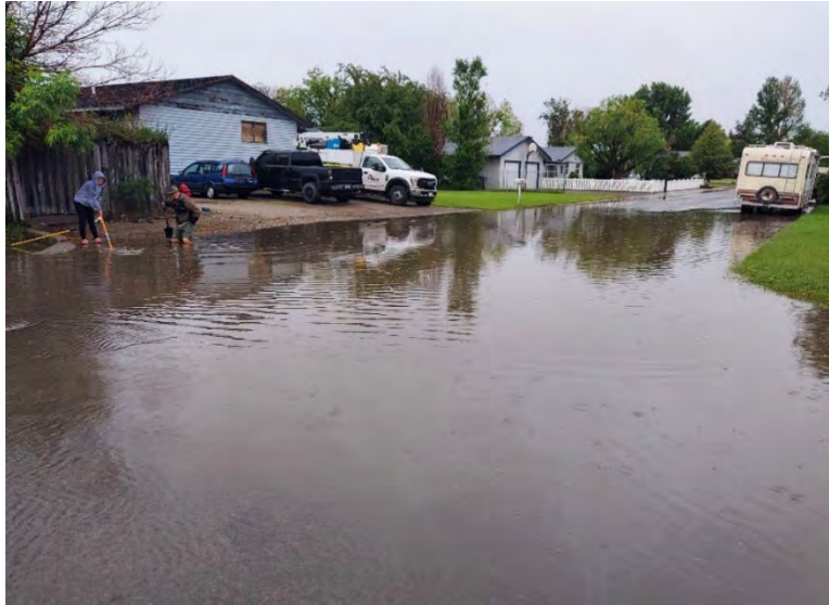
Photo 1: Ponding at Buffalo Road and Cougar Drive at Primary Outfall
