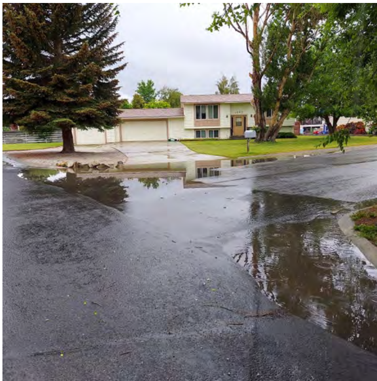
Photo 6: Flooding at Kodiak Road and Red Fox Drive
