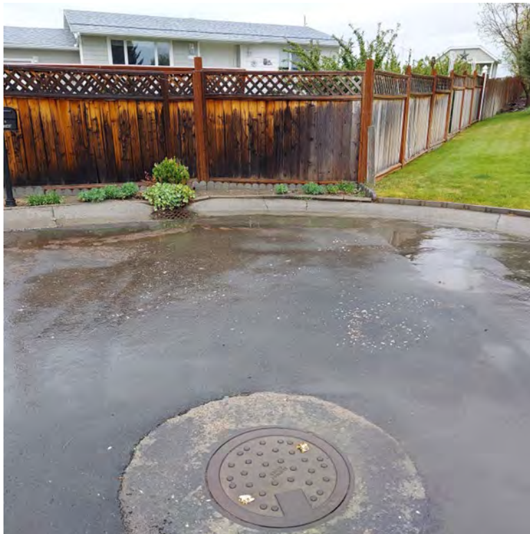
Photo 8: Flooding at Bighorn Road and Cougar Drive
