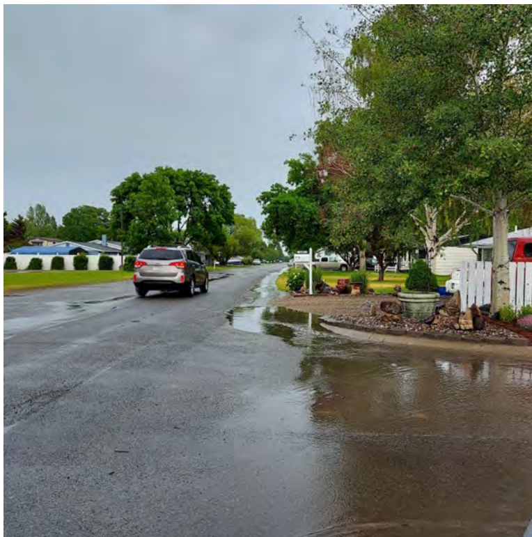
Photo 4: Flooding at Buffalo Road and Bobcat Drive
