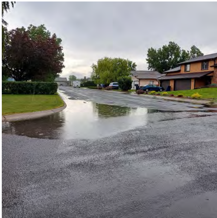
Photo 10: Flooding at Mustang Road and Wolverine Drive
