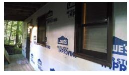
House Wrap (the white covering) was placed over the OSB. We are awaiting the delivery of the vinyl siding. As soon as it is received, the siding will be installed. We will also be taking down the railings on the first floor and reconstructing them to the building code. They will be higher, as the code is not 36" anymore, but 42" high. After the framing for the railings is complete, the cabling will be installed.
