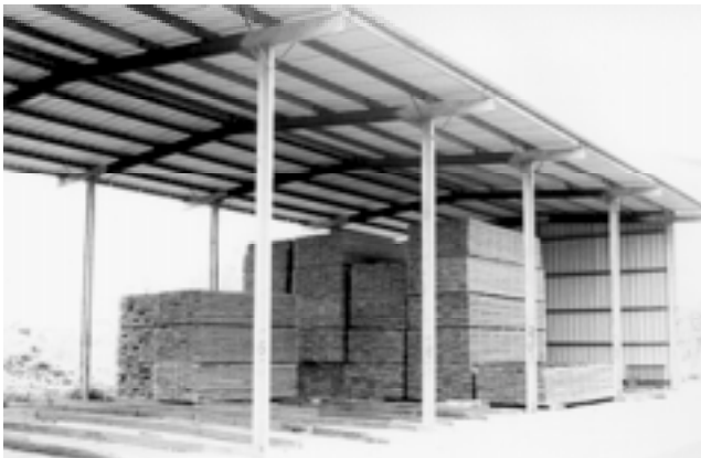
Figure 2—Shed for drying lumber protects the lumber from the weather.
