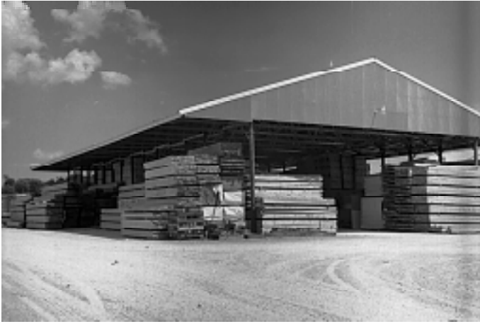
Figure 56—Open shed with louvered side wall helps protect lumber from wind-blown rain.
