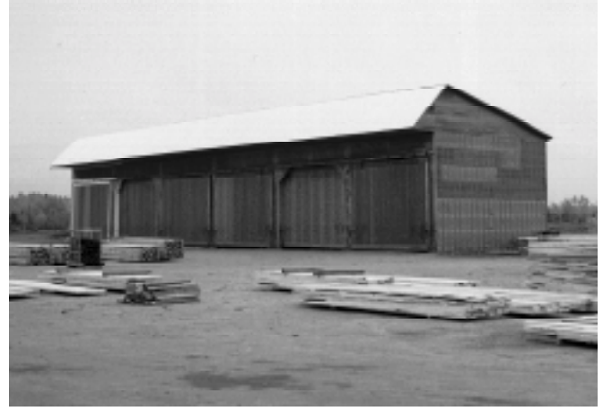
Figure 57—A closed, unheated lumber storage shed.
