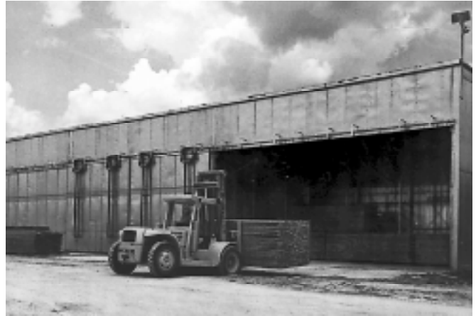
Figure 5—Typical package-loaded dry kiln.
