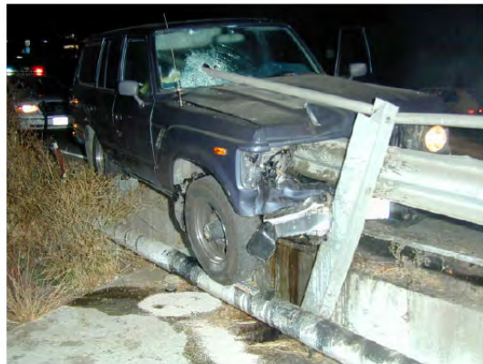
Figure 1. Example of “Knife Edge” Guard Rail Collision (Orcutt Road)
