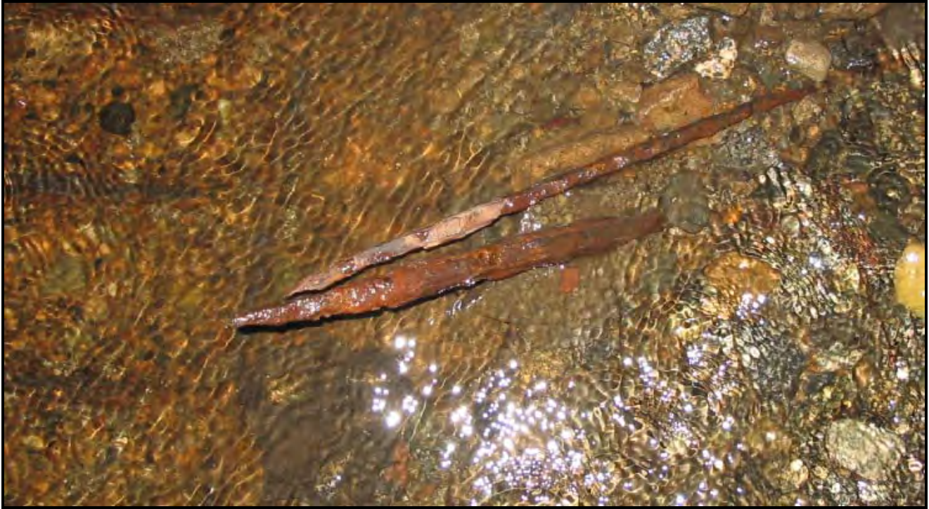
Garden Street Culvert Floor
