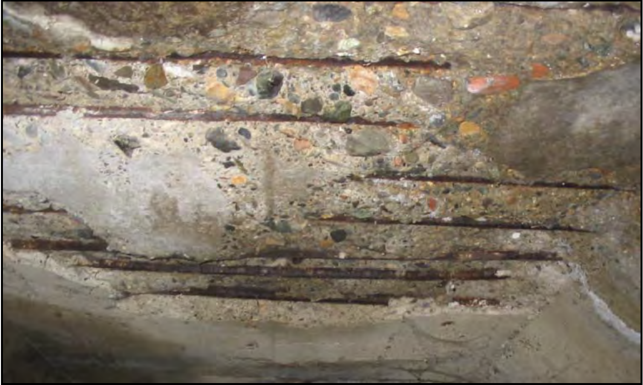
Garden Street Culvert Roof
