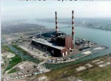
Trenton Channel - 730 mw
