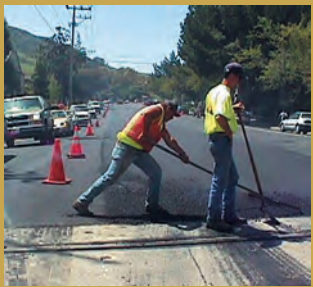
Repairing city streets and fixing potholes
