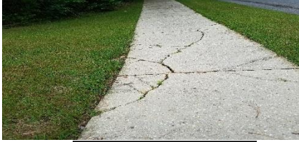
Cracked Sidewalk
