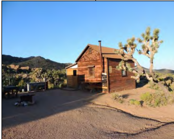
One of the buildings that has been refurbished
