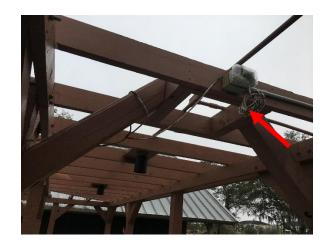
r. **Pavilions:** Recommend placing an outlet cover over the electrical socket place on pole under pavilion next to courts. As it could be an electrical hazard.
