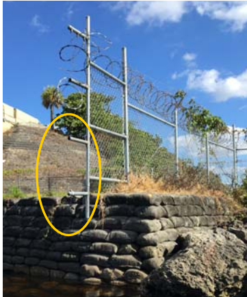
Razor wire has been removed.
