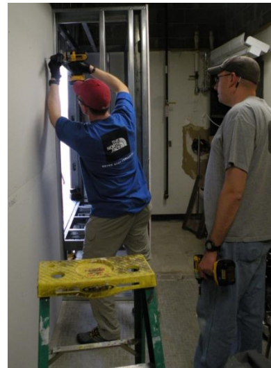
Captains Brian Clason and Jeremy Nichols installing drywall.
