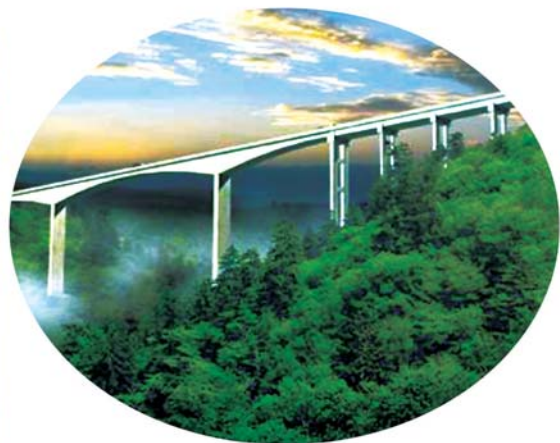
Rendering of Chipwi Bridge under construction
