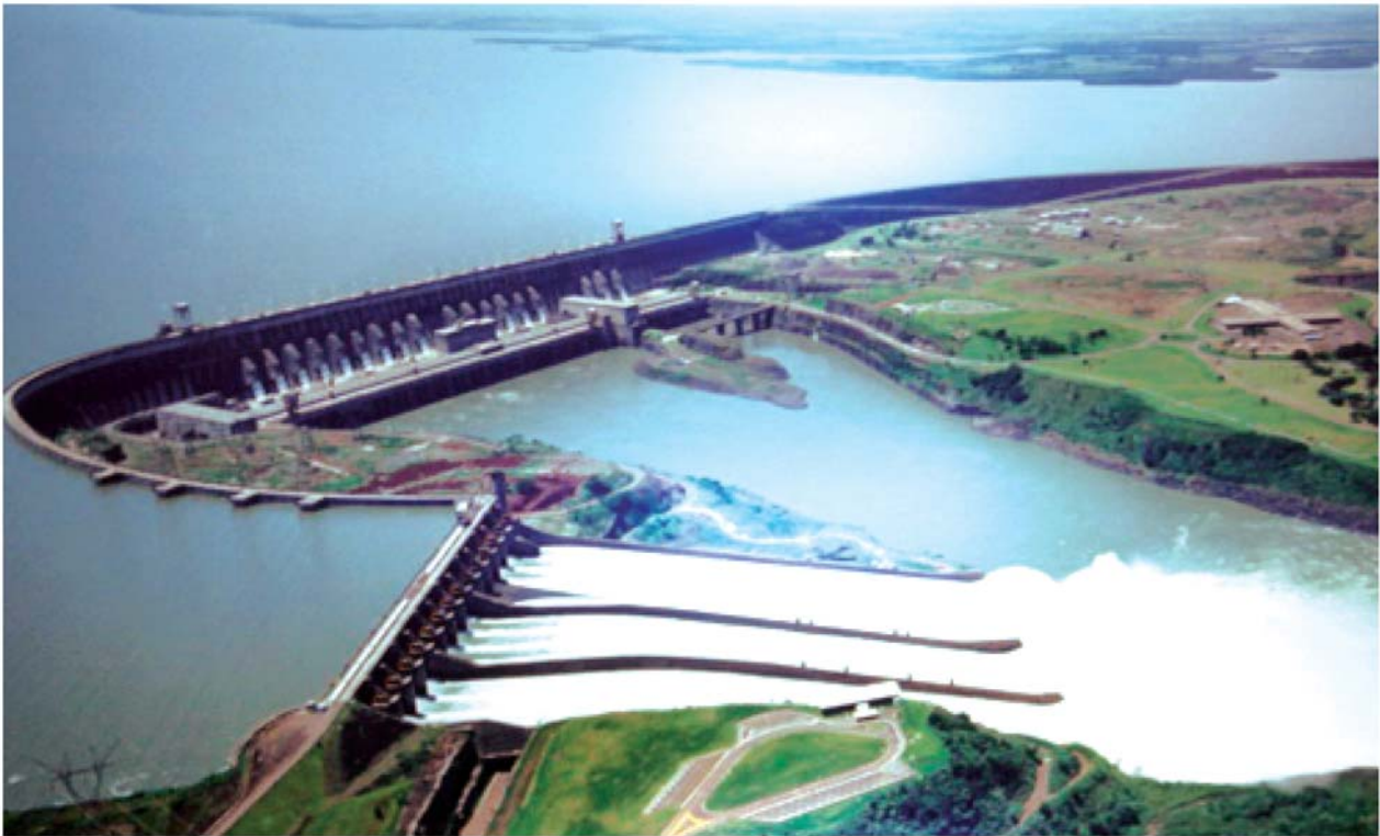
Itaipu Hydropower Station in Brazil and Paraguay, total installed capacity 14000MW, energy output 94.68 billion kWh in 2008, providing 90% of electricity consumed in Paraguay and 19% of that in Brazil
