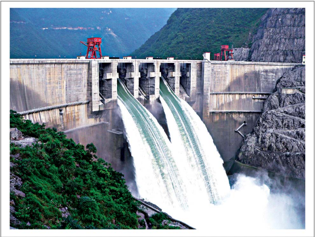
Hydropower Power Station
