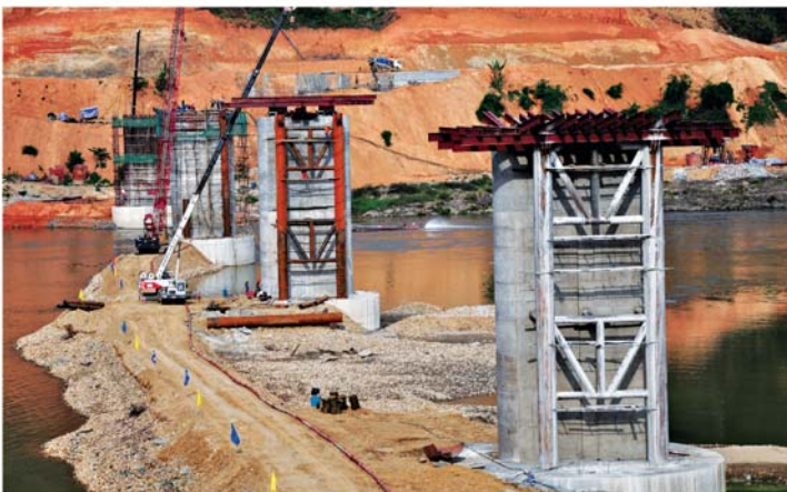
Myitsone Bridge under construction
