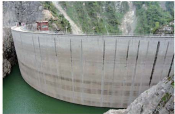
Shapai Dam (130m high, RCC arch dam)
