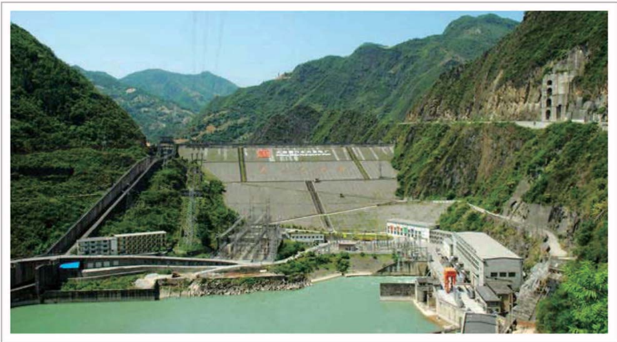
Bikou Dam (101m high, earth and rock dam)
