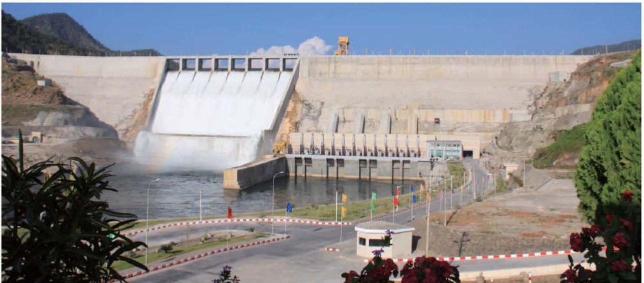
Yeywa Hydropower Station in Myanmar
