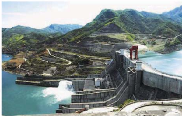
Baozhusi Dam (132m high, concrete gravity dam)
