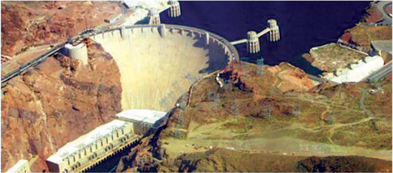
Hoover Hydropower Station in the USA, dam height 221m, installed capacity 2080MW, with flood-control, irrigation, water supply to city, and other comprehensive benefits
