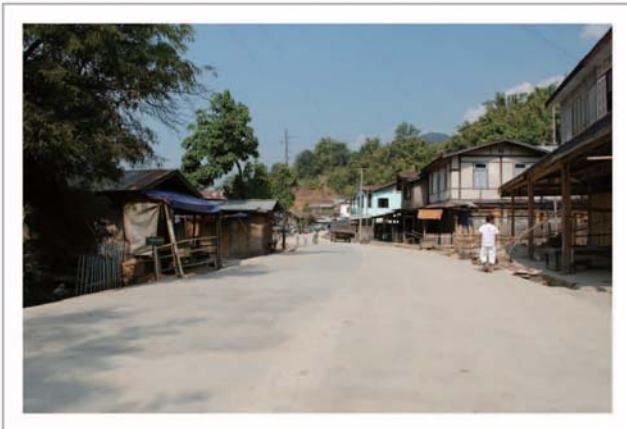
Upgraded Chipwi Road
