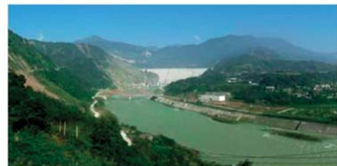
Zipingpu CFRD Dam Overview after Earthquake (156m high)
