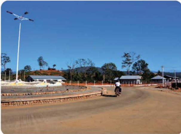
19.68 km new concrete road built in resettlement village, with free power and water supply to community
