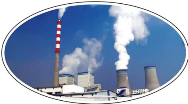
Coal-fired Power Plant
