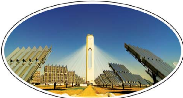
Solar Power Plant
