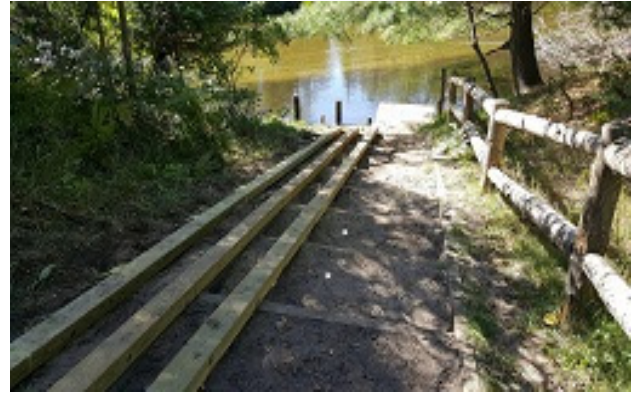
Three Mile Landing - After
