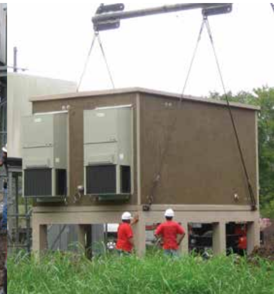
Placing the Building
