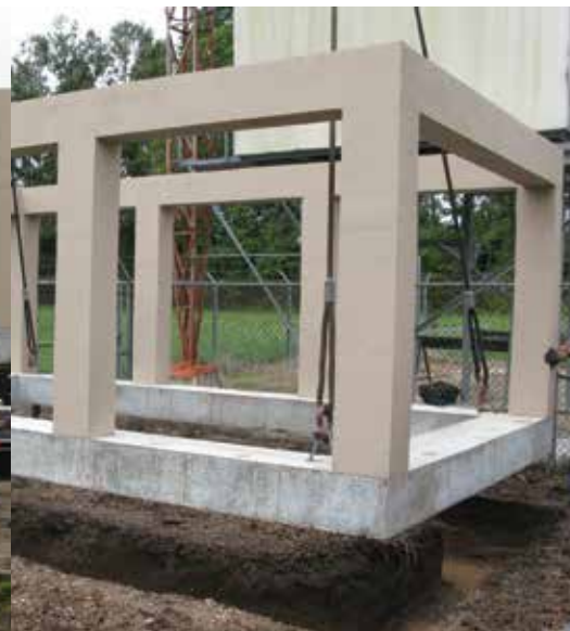
Placing the Chain Wall
