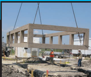
Chain Wall Installation
