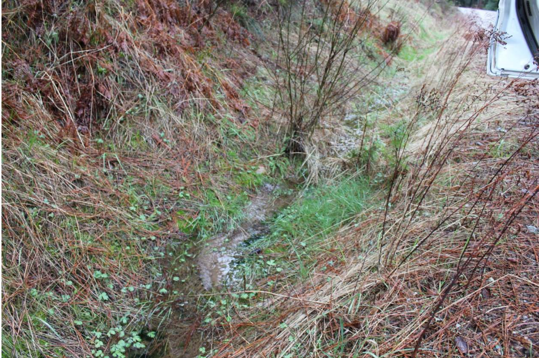
Figure 25: Roadside ditch intercepting and transmitting groundwater to Canyon Creek.
