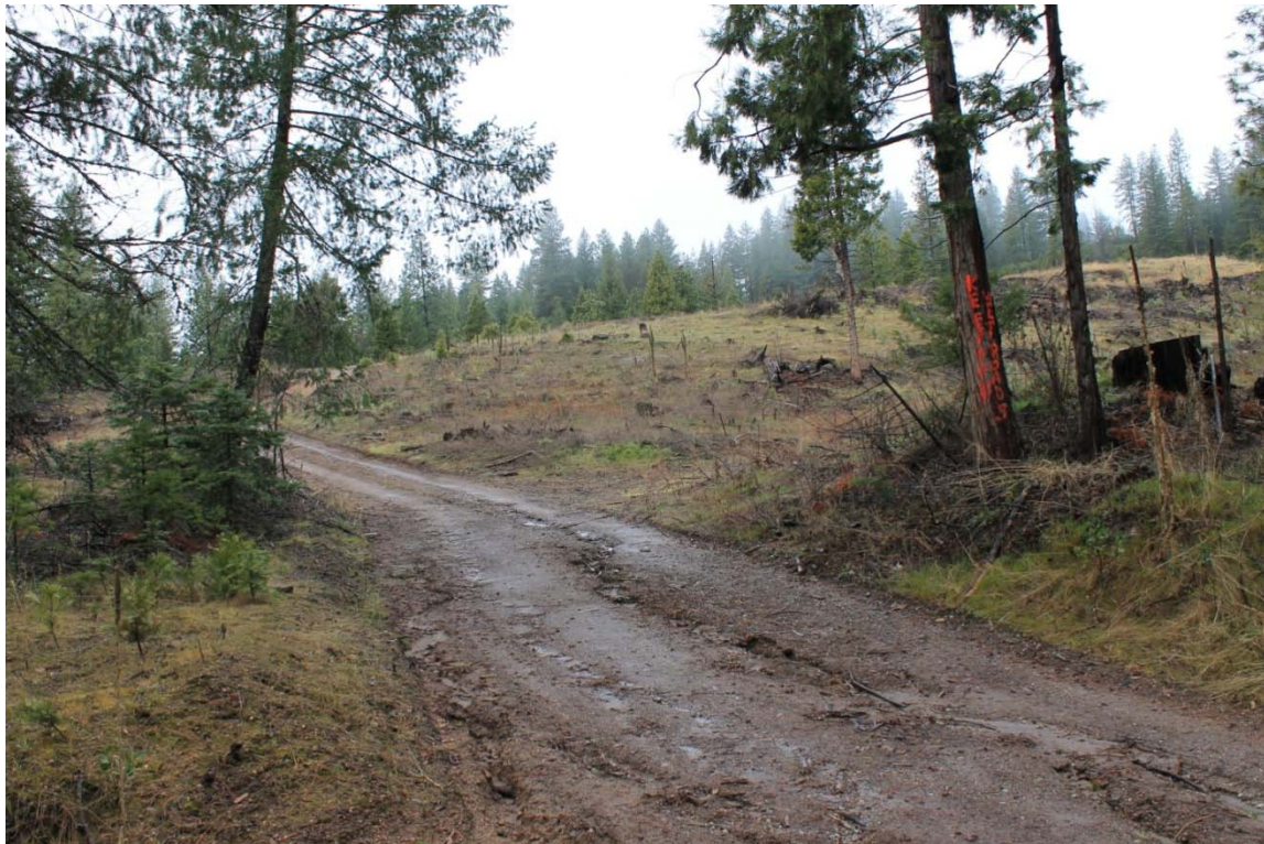
Figure 28: Gullies in road from clear cut in the Canyon Creek drainage.
