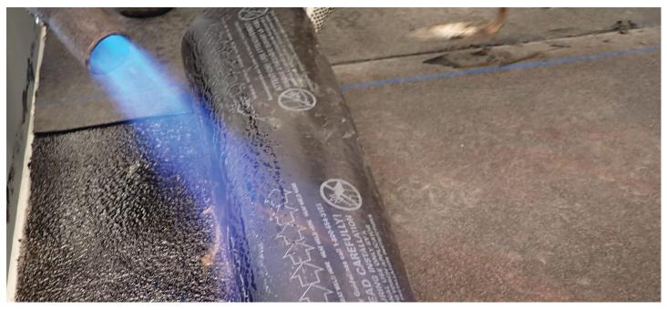
Photo 2: A view of the SBS polymer-modified bitumen base sheet being torched to a primed concrete deck during the roof system installation
