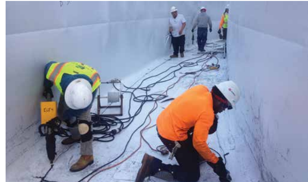
PHOTO 4 Welding crews performing extrusion welds.
