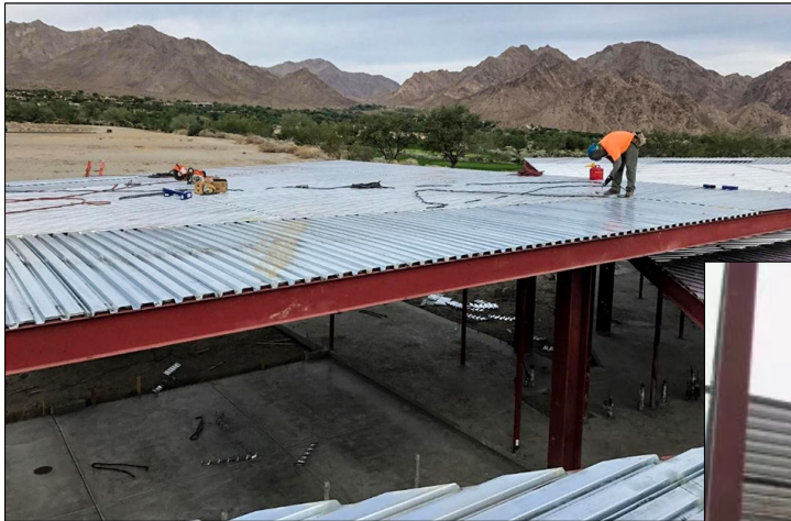
Steel roof deck
