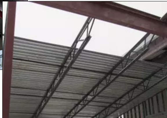
Steel roof deck on steel joists on steel beams
