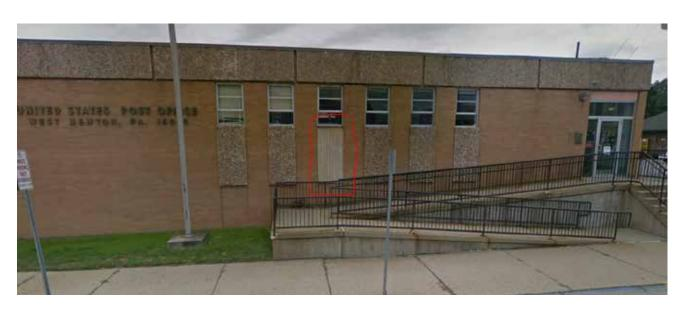
It was noticed that a section of the rock overlay was removed and replaced with plywood. The landlord confirmed they hadn't made this alteration and it was most likely completed by the USPS.
