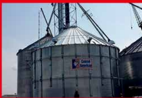
Grain Bin Construction and Remodeling
