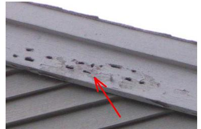
6. General overview of exterior. Exterior Surface Corner boards **NOTE: Sections of DAMAGED corner boards due for correction.**
