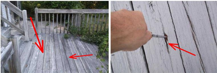
11. REAR DECK Deck / Porch Railings NOTE: The railing guards are HORIZONTAL and have a ladder effect which is normally not allowable, question Contractors and correct if and as needed.
