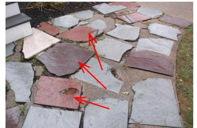
3.           Exterior steps/stoop/landing. (Not attached to Deck or Porch.) NOTE: LOOSE TREADS due for correction.
