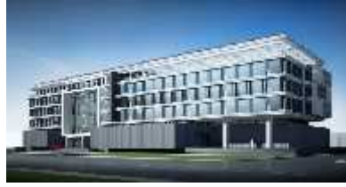
Commercial & Public Buildings
