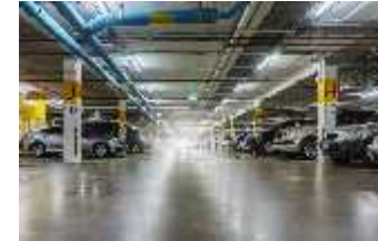
Enclosed Vehicular Facilities
