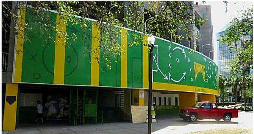
124' x 10' TS22 frame - Rowdies Soccer Stadium in St Pete, FL.
