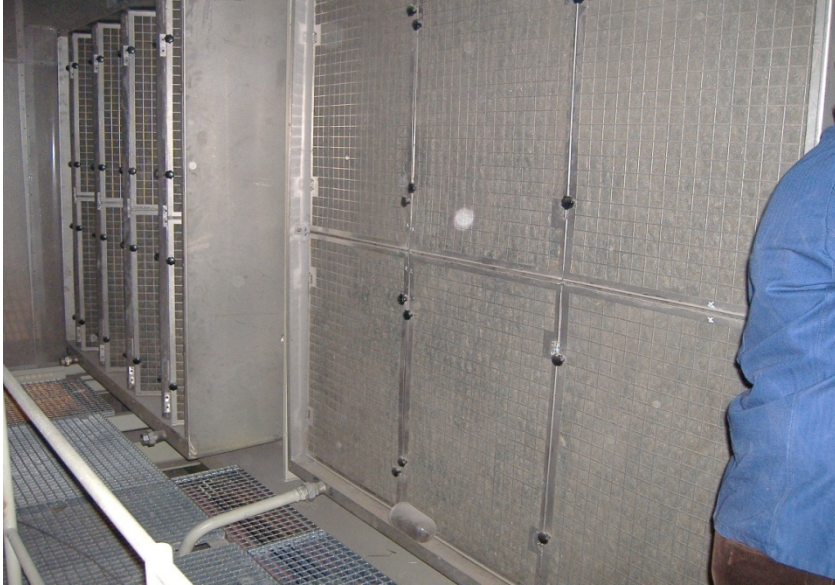
DCF 2 (left) and DCF 1 (right) Quick-opening device for filter-change
