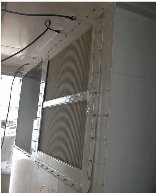
DFH installed in the intake section for engine room ventilation
