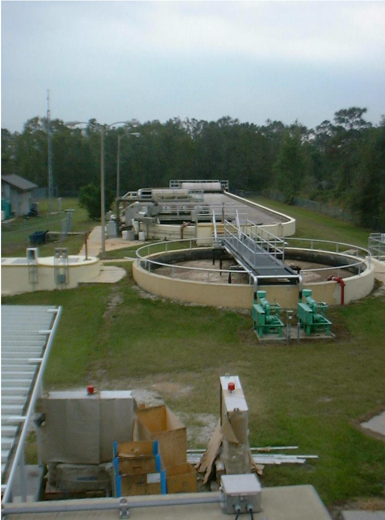
Figure 5.1 - WWTP 1 Oxidation ditch and converted sludge thickener
