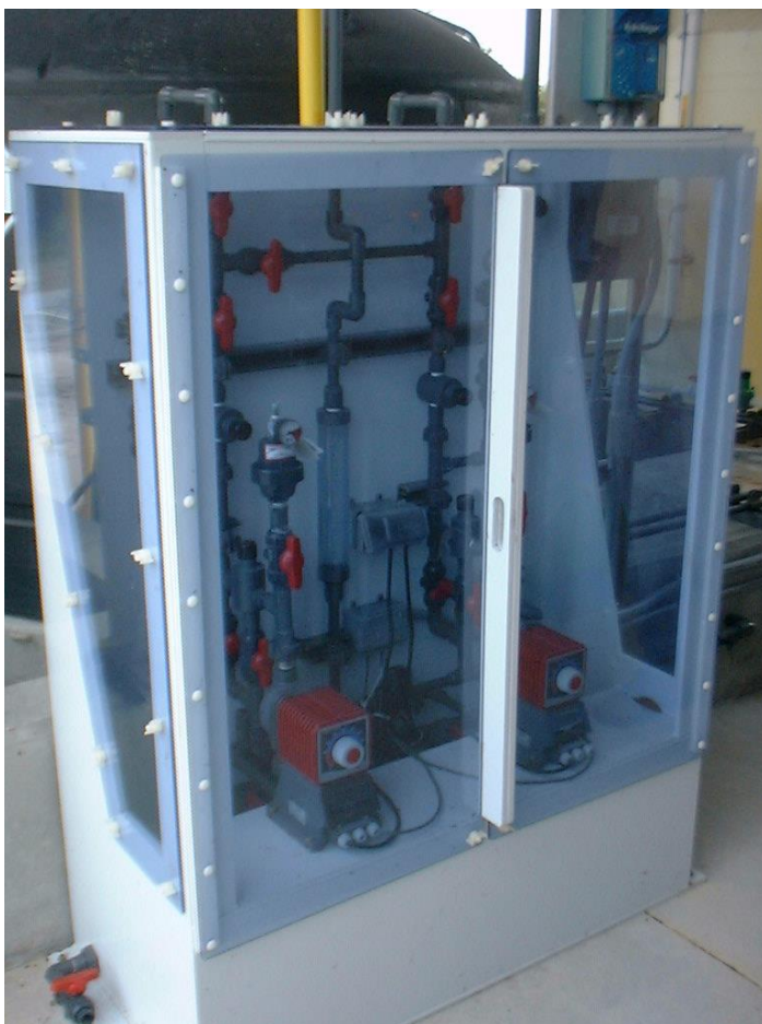
Figure 5.24 – New WWTP 3 Sodium Hypochlorite feed and control system. Note this is typical for all Poinciana hypochlorite facilities
