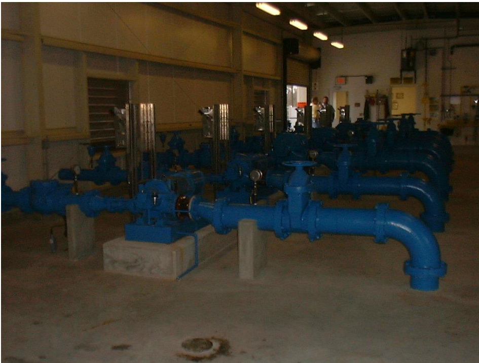
Figure 4.31 - New high service pumping room at WTP 5
