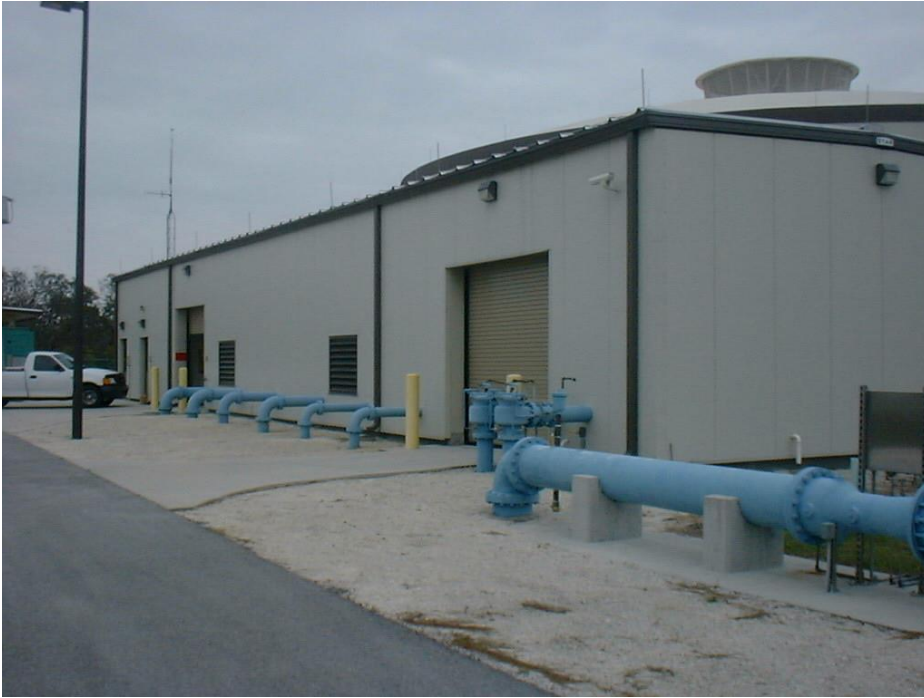
Figure 4.30 - New Ops building WTP 5 that houses the high service pumps (6 pipes from high service pumps visible in photograph)
