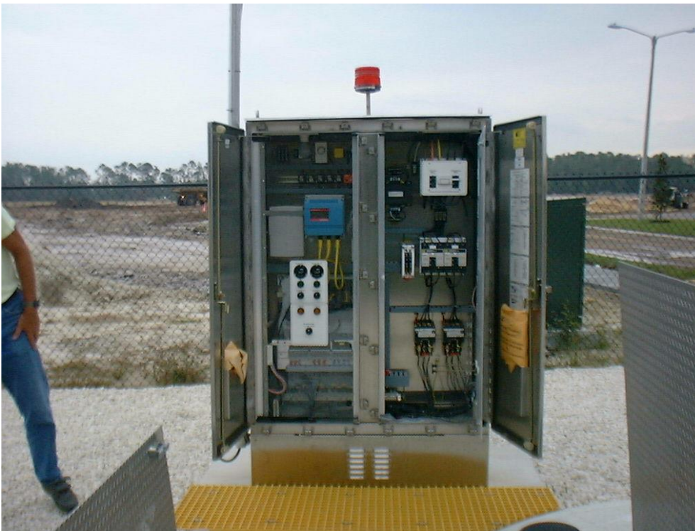
Figure 7.6 - New Lift station control box open
