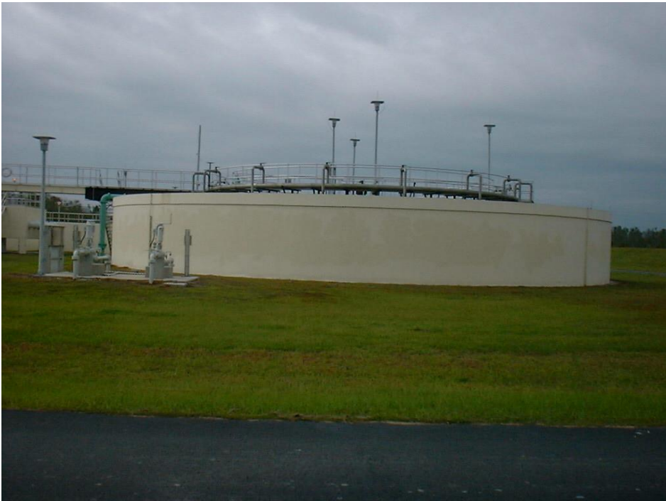
Figure 5.13 - WWTP 2 clarifiers (converted from old aeration basins)
