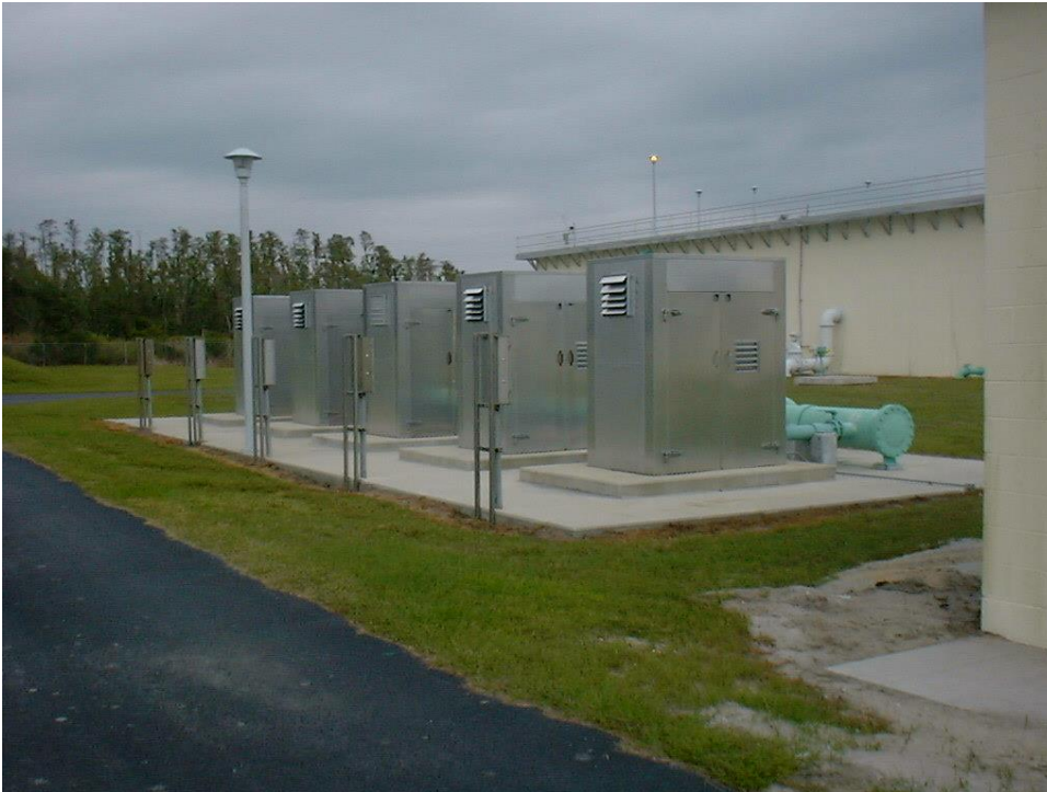
Figure 5.9 – New WWTP 2 Blowers for SBR facility (located in background)
