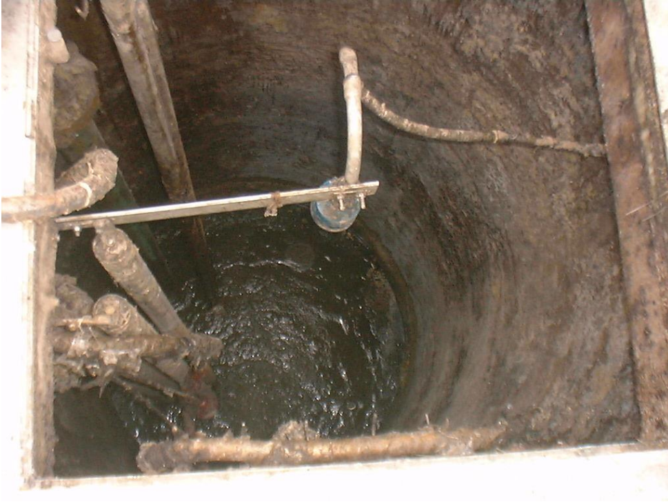
Figure 7.1 – Typical Lift Station Wet well
