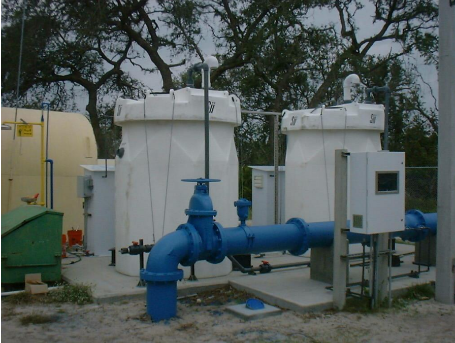
Figure 4.24 – New sodium hypochlorite system at WTP 4. Old WTP 4 aerator and hydropneumatic tank shown in background (to be abandoned)
