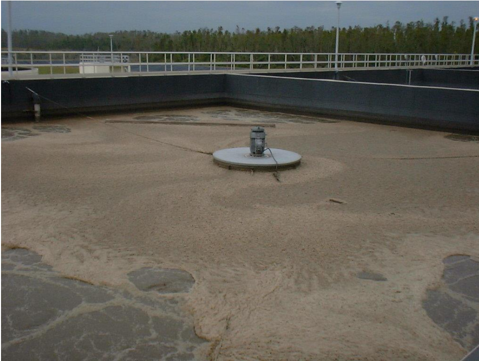
Figure 5.11 - WWTP 2 SBR – typical of 4 basins
