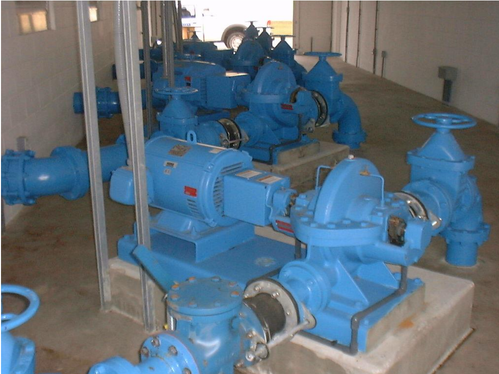
Figure 4.35 – High service pumps for WTP 6. Note that only 3 of 5 possible pumps are installed (see Figure 4.36)
