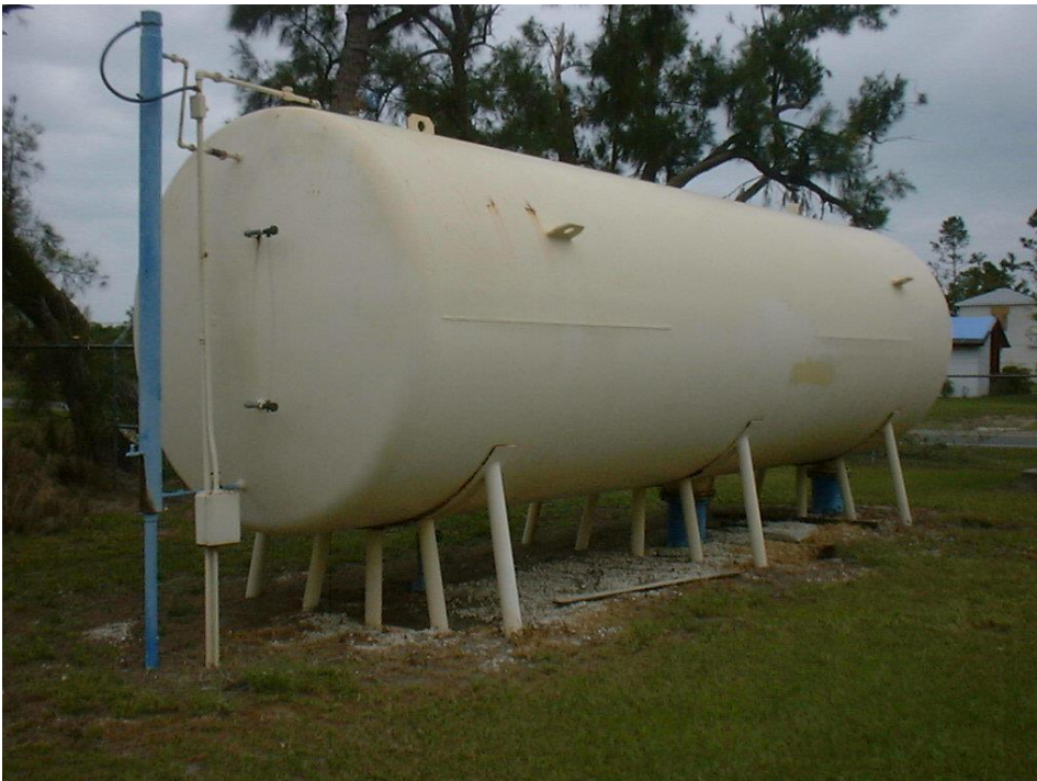
Figure 4.19 – 10,000 gallon hydropneumatic tank at WTP 3
