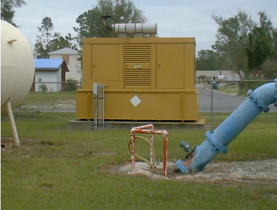
Figure 4.20 WTP 3 Generator with belly tank at WTP 3 site. Hydropneumatic tank and finished water line from pump system shown on the edges of photograph.
