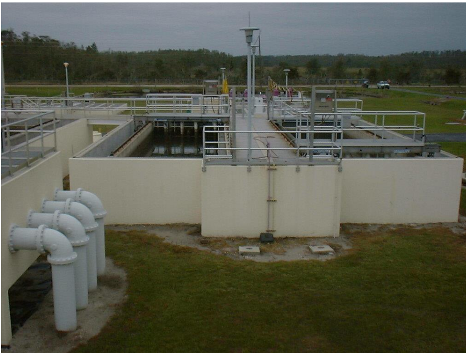
Figure 5.14 – New WWTP 2 Traveling Bridge Filter
