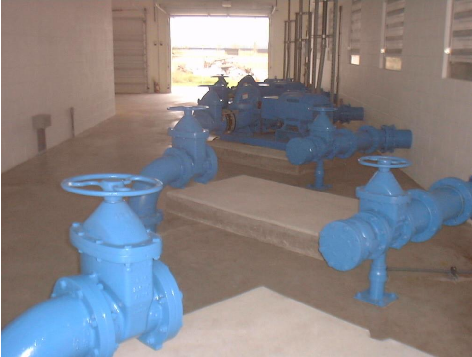
Figure 4.36 – Room for additional pumps in High service pumping facility at WTP 6
