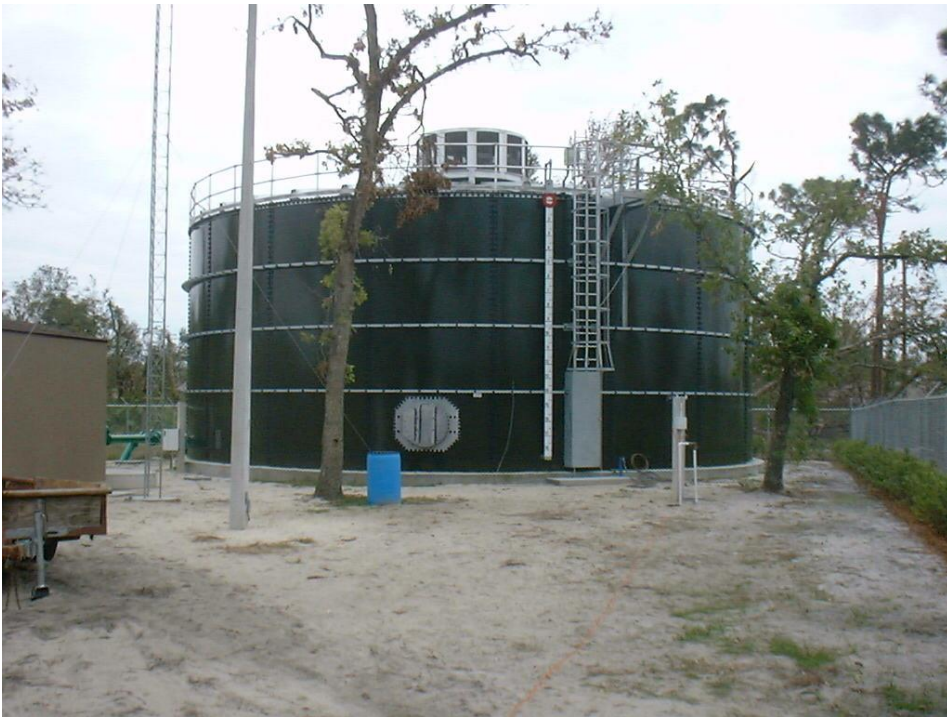
Figure 4.23 - New Glass lined 250,000 gallon tank and new aerator at WTP 4 – not in service as of December 2004.
