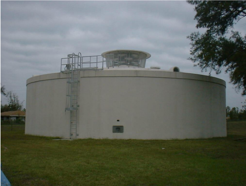
Figure 4.18 - 350,000 gallon storage tank and aerator at WTP 3
