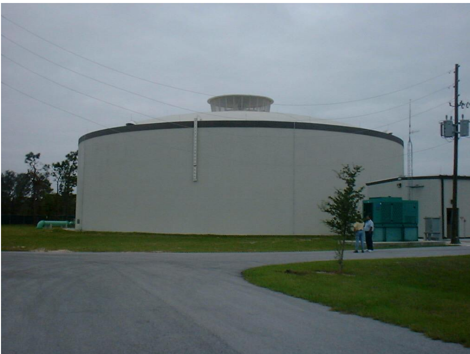
Figure 4.27 - New one million gallon storage tank with aerator at WTP 5. Diesel generator and high service pumping building at right side of photograph)
