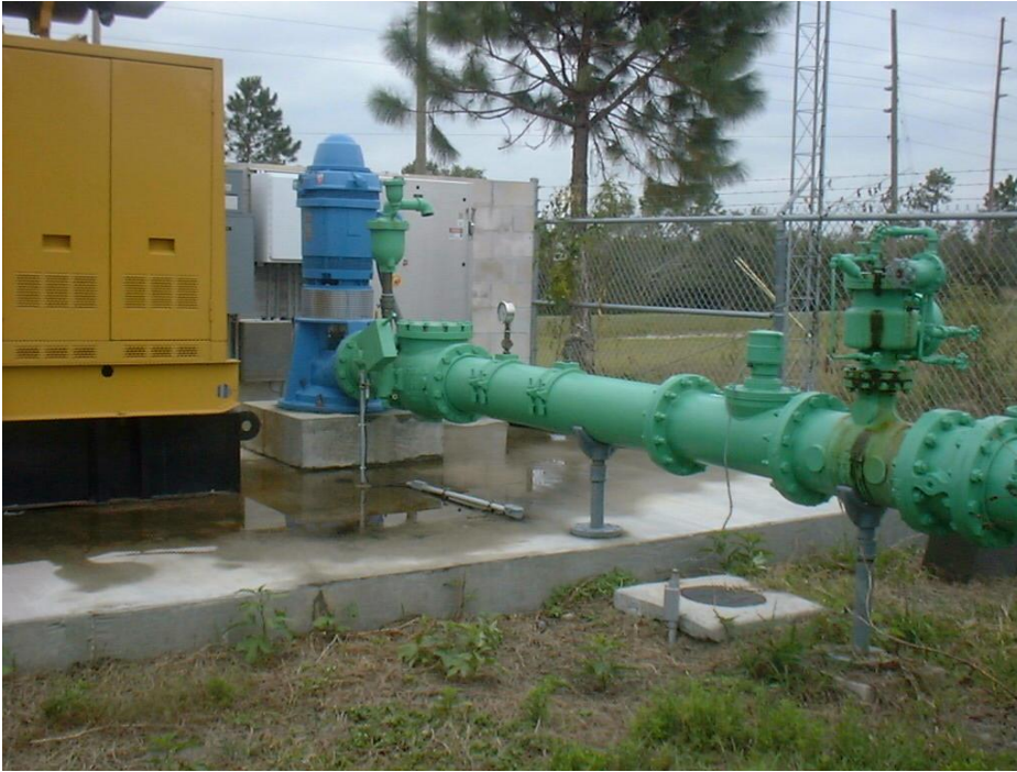
Figure 4.26 - New 2400 gpm well to provide raw water to WTP 5 located off-site. A generator is provided for this facility
