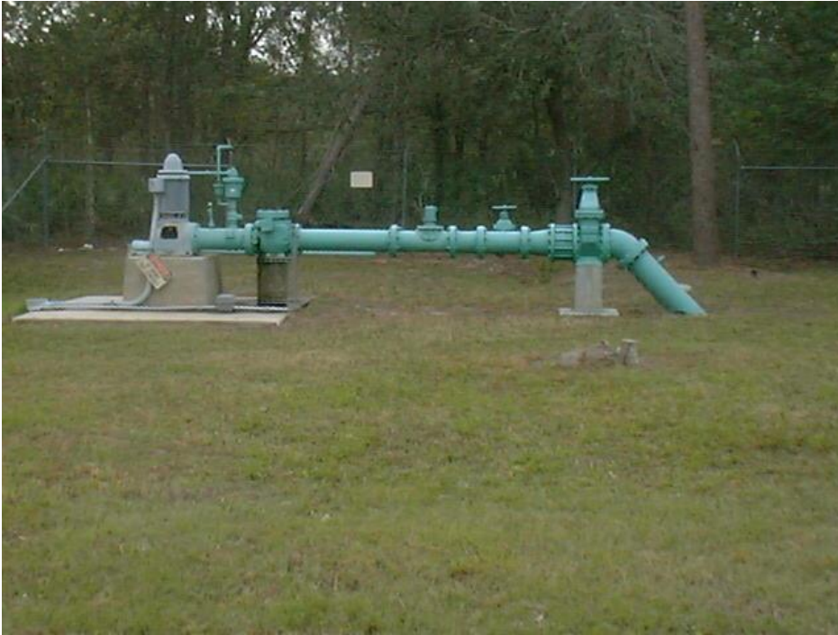
Figure 4.4 - Well at WTP 1 off site. This well is in an industrial park with no wellhead protection measure.
