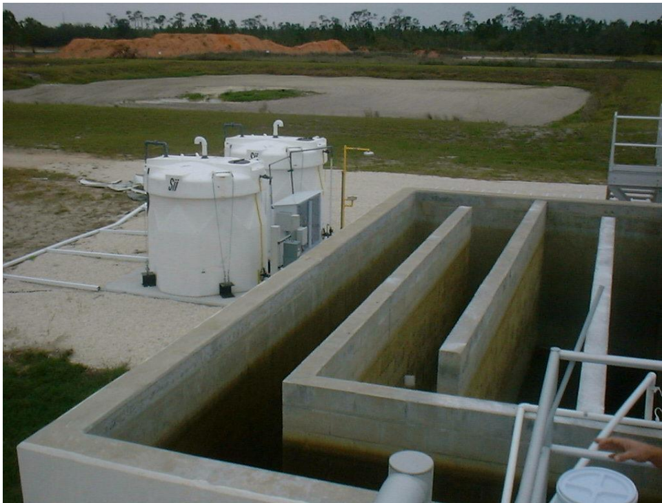
Figure 5.32 - New Chlorine contact chamber at WWTP5 and sodium hypo system
