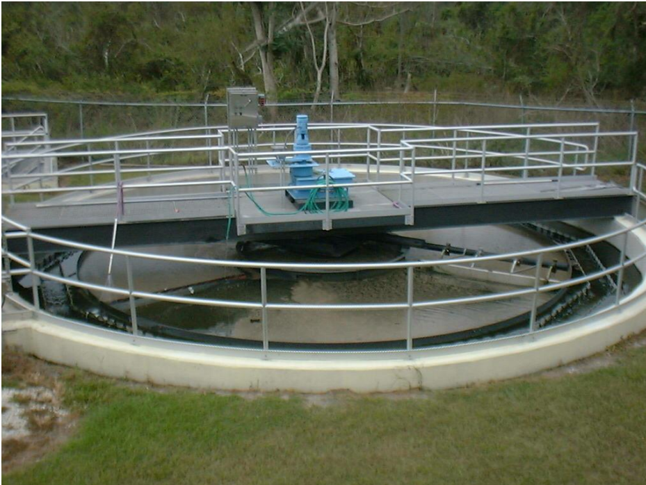
Figure 5.2 – New WWTP 1 Clarifiers. The old clarifier now used as a thickener at left.
