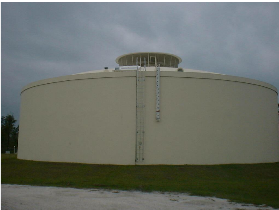
Figure 4.32 – 500,000 gallon storage tank and aerator for WTP 6
