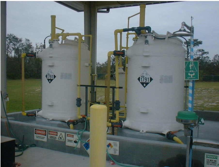
Figure 4.29 – New sodium hypochlorite system at WTP 5
