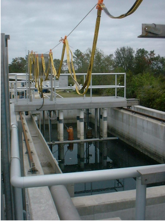
Figure 5.22 – New WWTP 3 Traveling Bridge Filter
