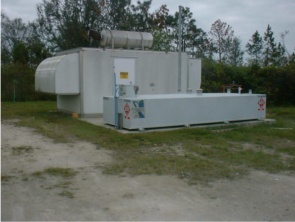
Figure 5.25 – New WWTP 3 Generator
