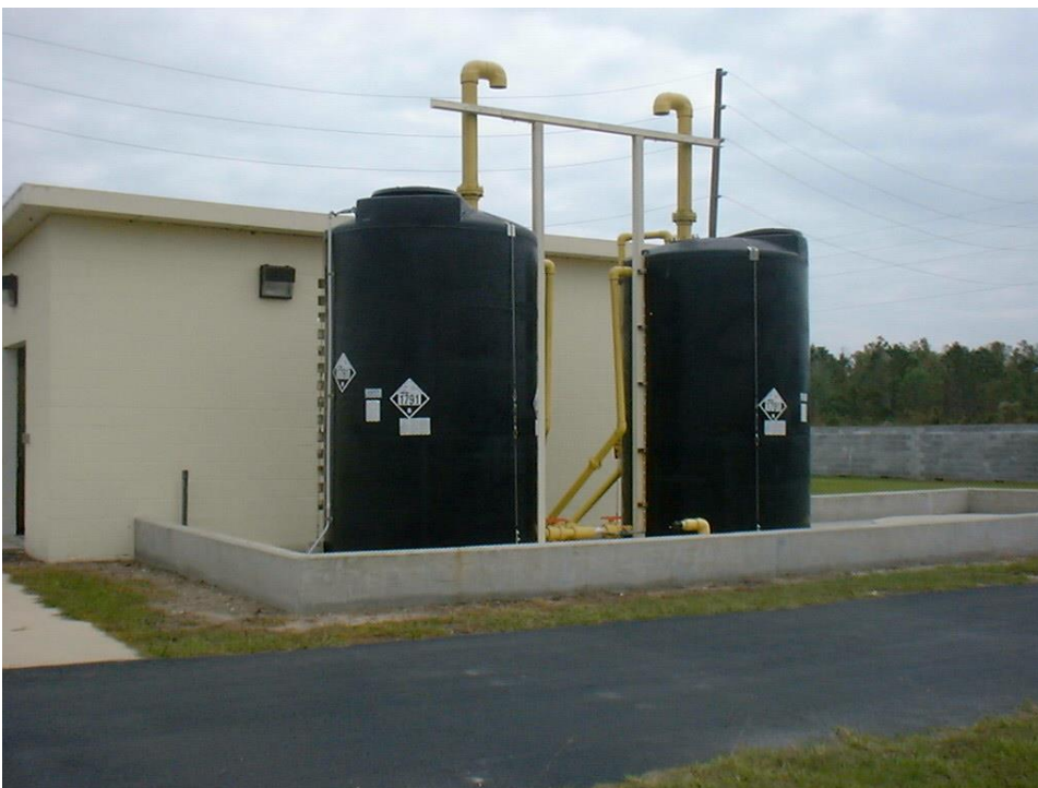
Figure 5.18 – New WWTP2 Sodium Hypochlorite system
