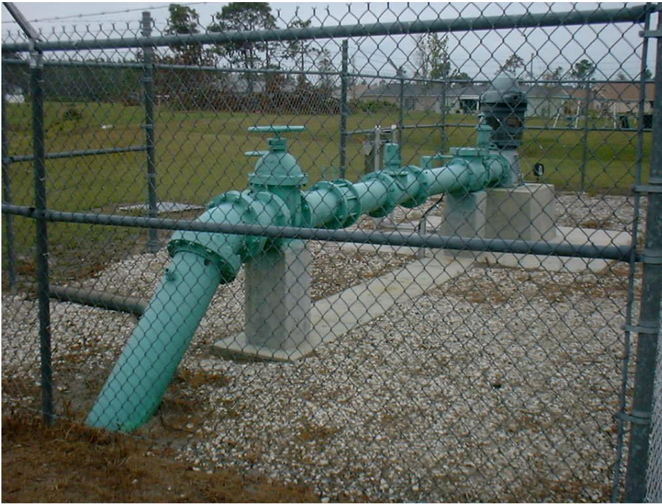
Figure 4.10 – One of the water supply wells for WTP 2 located off the plant site.
