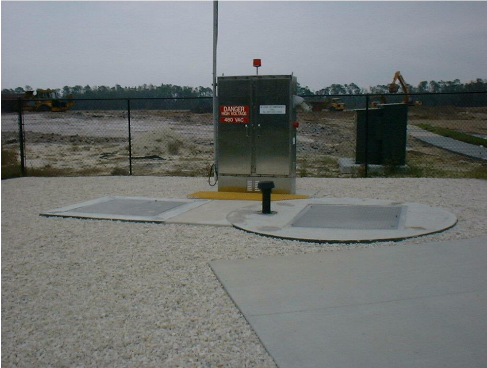
Figure 7.5 - New lift station installation
