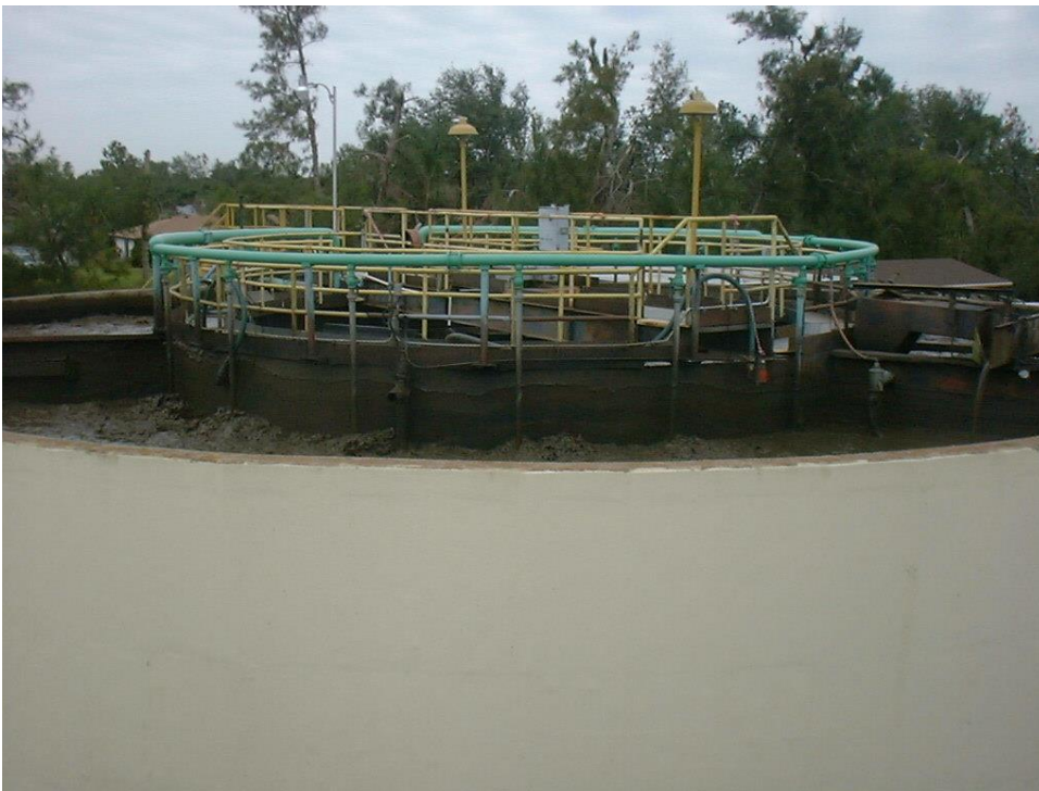
Figure 5.26 - Old WWTP 3 converted to digester
