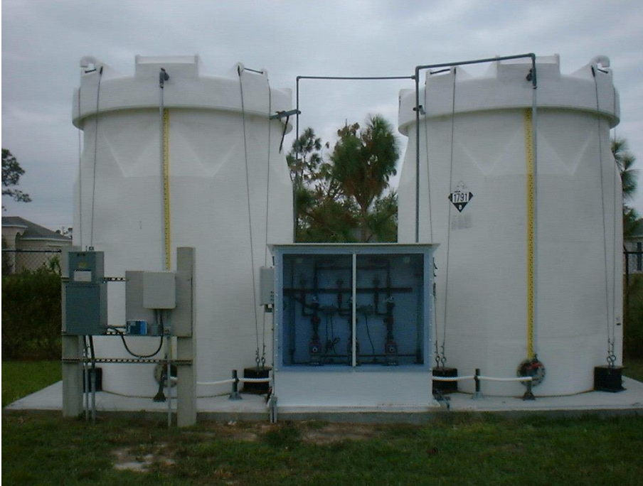
Figure 4.14 - WTP 2 Sodium hypochlorite system
