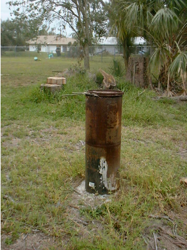
Figure 4.16 - WTP 3 uncapped well casing
