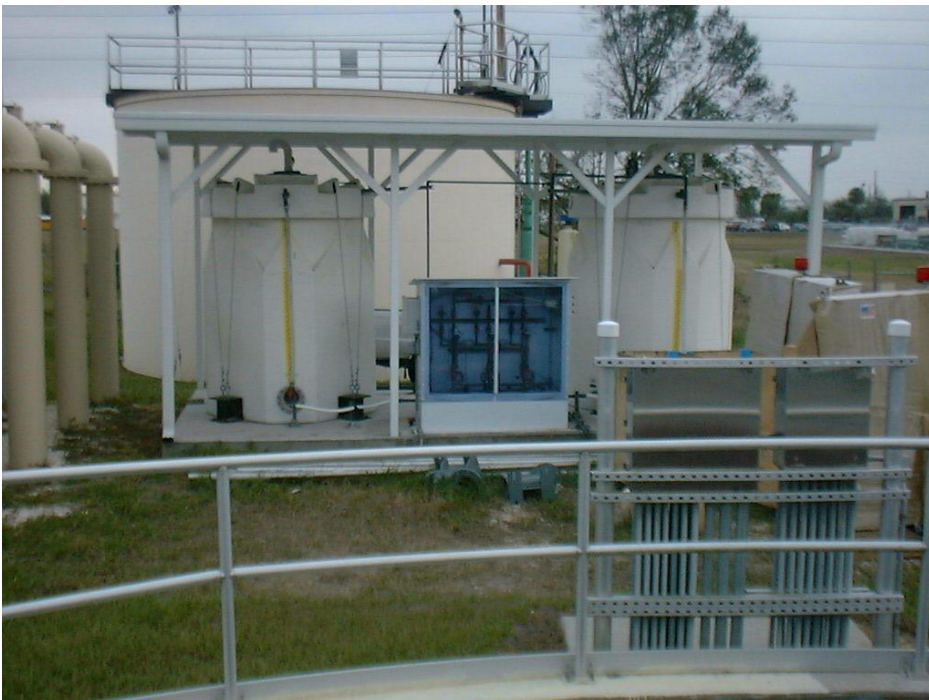
Figure 5.5 - Sodium Hypochlorite system at WWTP 1
