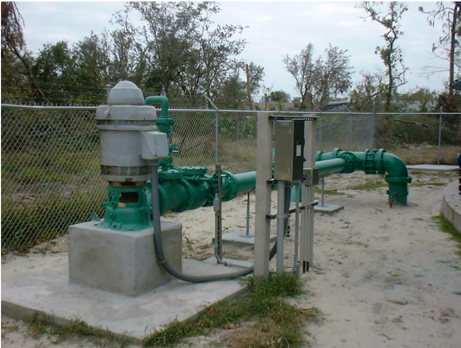
Figure 4.22 –1000 gpm well fire well with new sanitary seal and pump based at WTP 4
