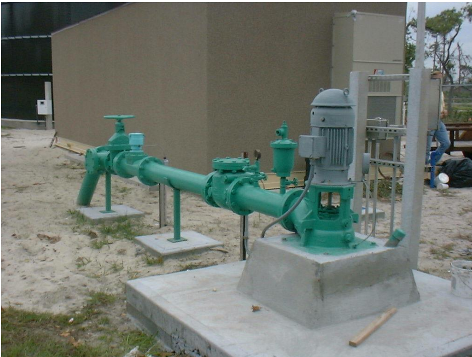
Figure 4.21 – New well sanitary steel and pump base for 300 gpm well on the site of WTP 4. New glass-lined steel tank and new electrical/mechanical control building shown behind well
