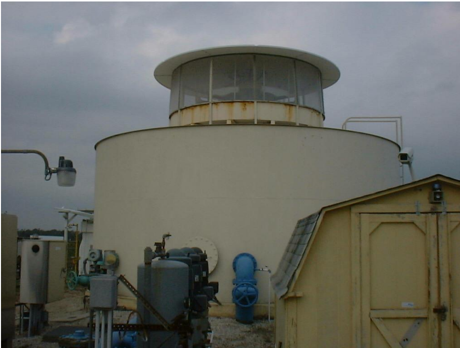
Figure 4.6 – 50,000 gallons storage tank and aerator at WTP no. 1. The aerator does not appear to have been upgraded to match the plant capacity.
