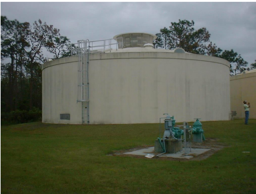
Figure 4.13 – Newer 600,000 gallon tank and aerator at WTP 2 new tank and on-site well
