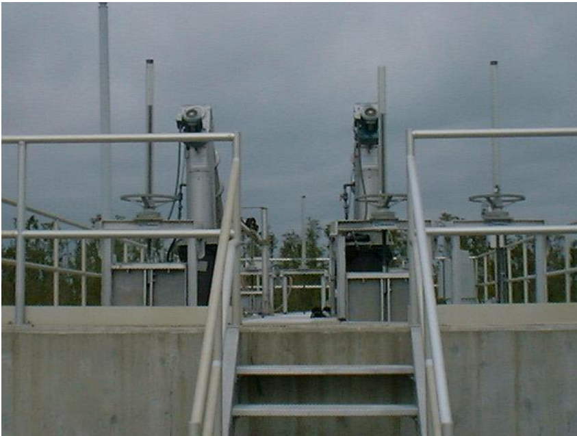
Figure 5.8 – New WWTP 2 Influent screw pumps
