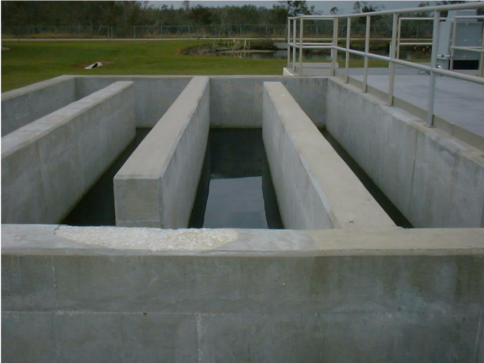
Figure 5.15 – New WWTP 2 Chlorine Contact Chamber
