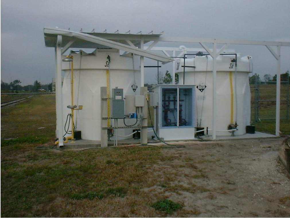
Figure 4.8 – New WTP 1 Sodium Hypochlorite system. Damage to roof caused by Hurricane in the fall of 2004 and will be repaired shortly.
