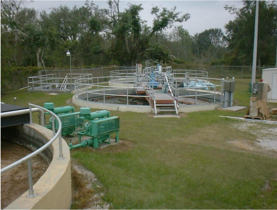
Figure 5.2 – New WWTP 1 Clarifiers. The old clarifier now used as a thickener at left.
