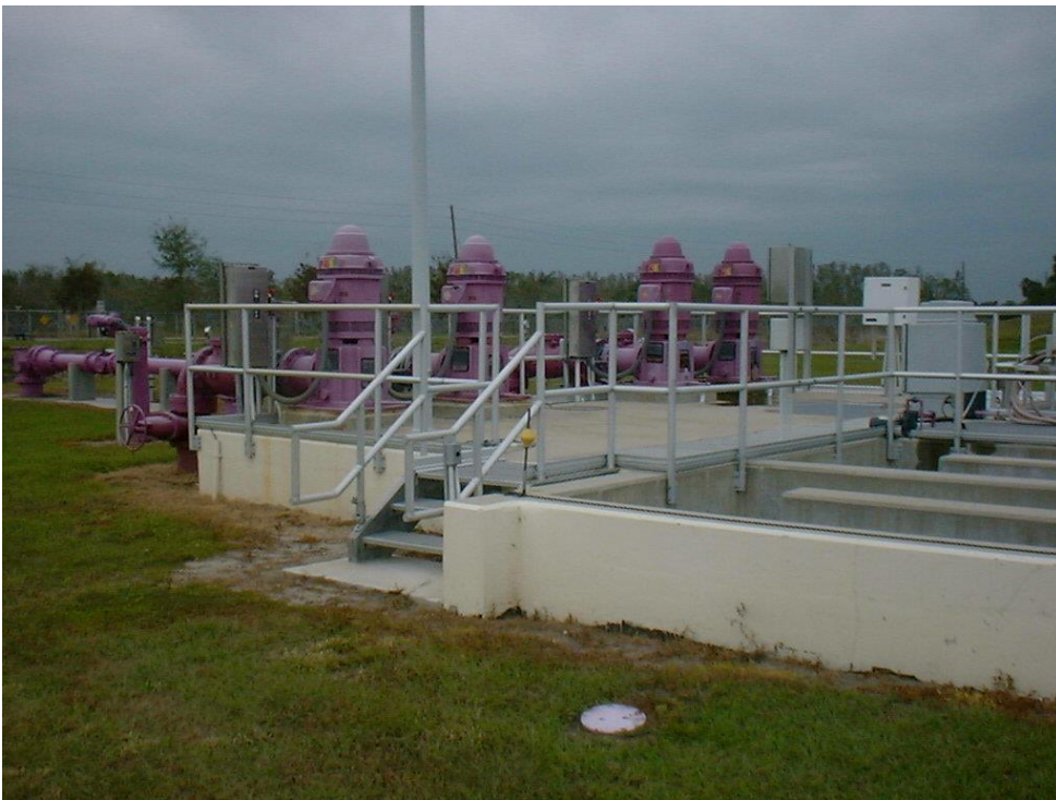
Figure 5.16 - WWTP 2 Chlorine Contact Chamber and Reuse Pumps
