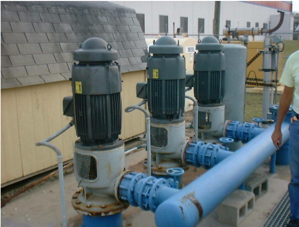
Figure 4.7 - WTP 1 high service pumps (3 – 20 hp motors)
