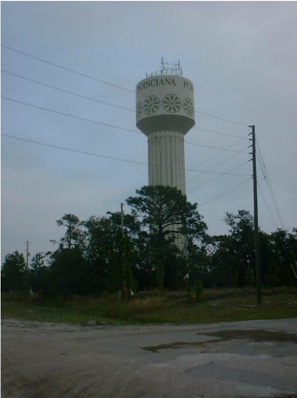
Figure 4.3 - Offsite 400,000 gal elevated tank. A series of cell phone towers have been added to the tank since 1999 which is a source of revenue for the system. If other elevated tanks are considered for fire protection purposes, these aerials should be considered for co-location..
