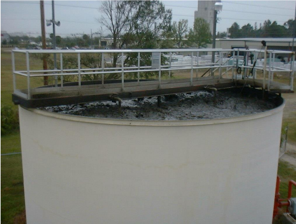
Figure 5.6 – WWTP 1 Sludge thickener
