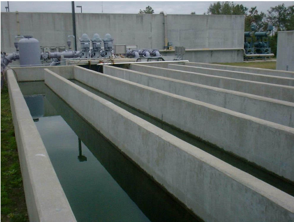
Figure 5.23 – New WWTP 3 Chlorine contact chamber
