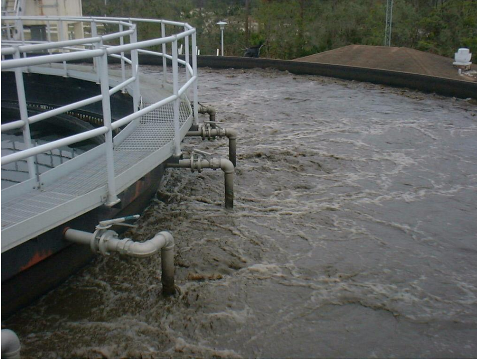
Figure 5.29 - WWTP Contact Aeration basin
