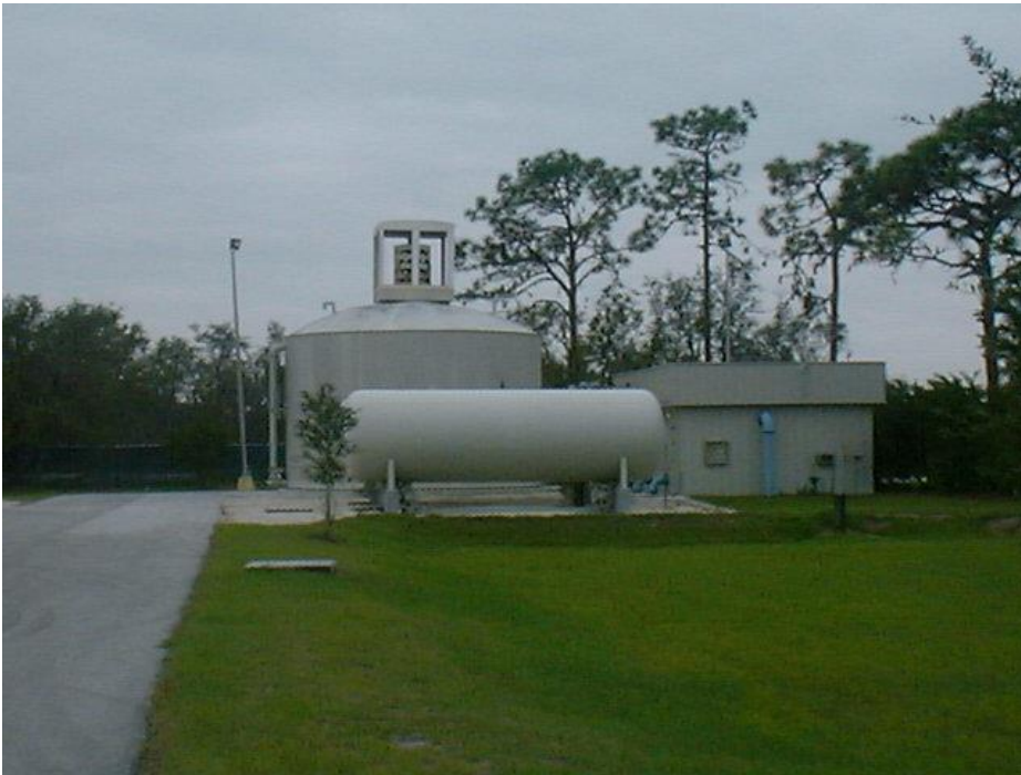
Figure 4.28- New hydro-pneumatic tank, old steel storage tank and old high service pump building at WTP 5. The old tank and pump building have been abandoned
