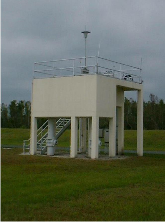
Figure 5.7 – WWTP 2 Headworks – expandable by replication to 6 MGD
