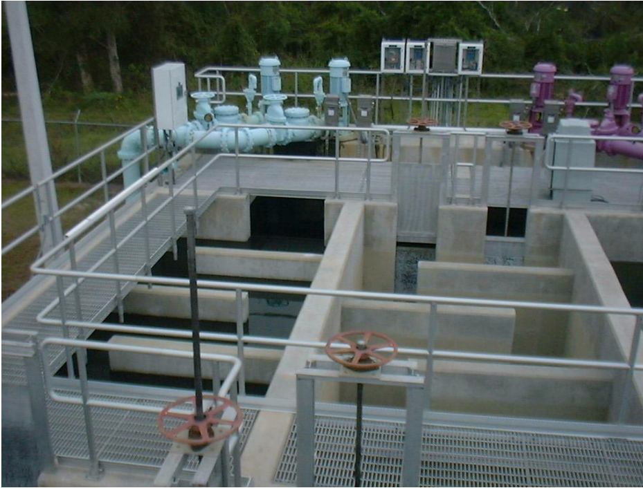
Figure 5.4 - WWTP 1 Chlorine contact chamber
