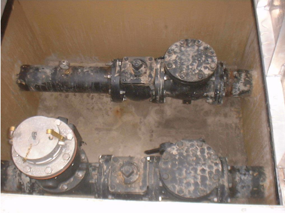
Figure 7.7 - New Lift station valve vault
