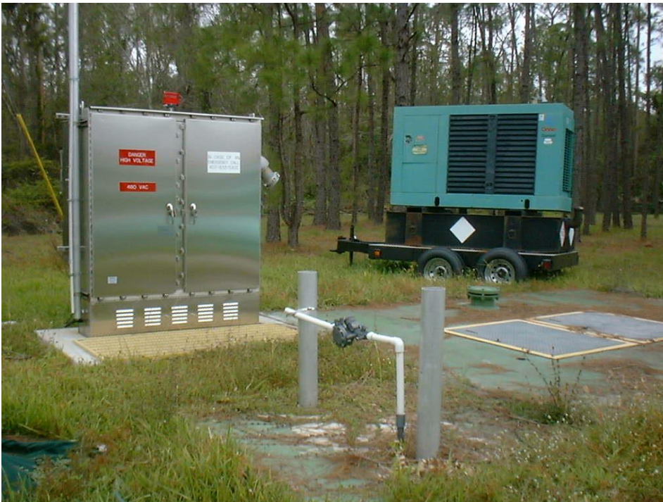
Figure 7.4 - Typical Lift station with portable generator
