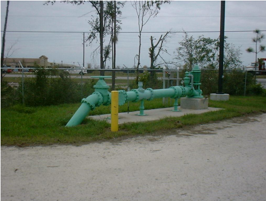
Figure 4.31 – New well to service WTP 6
