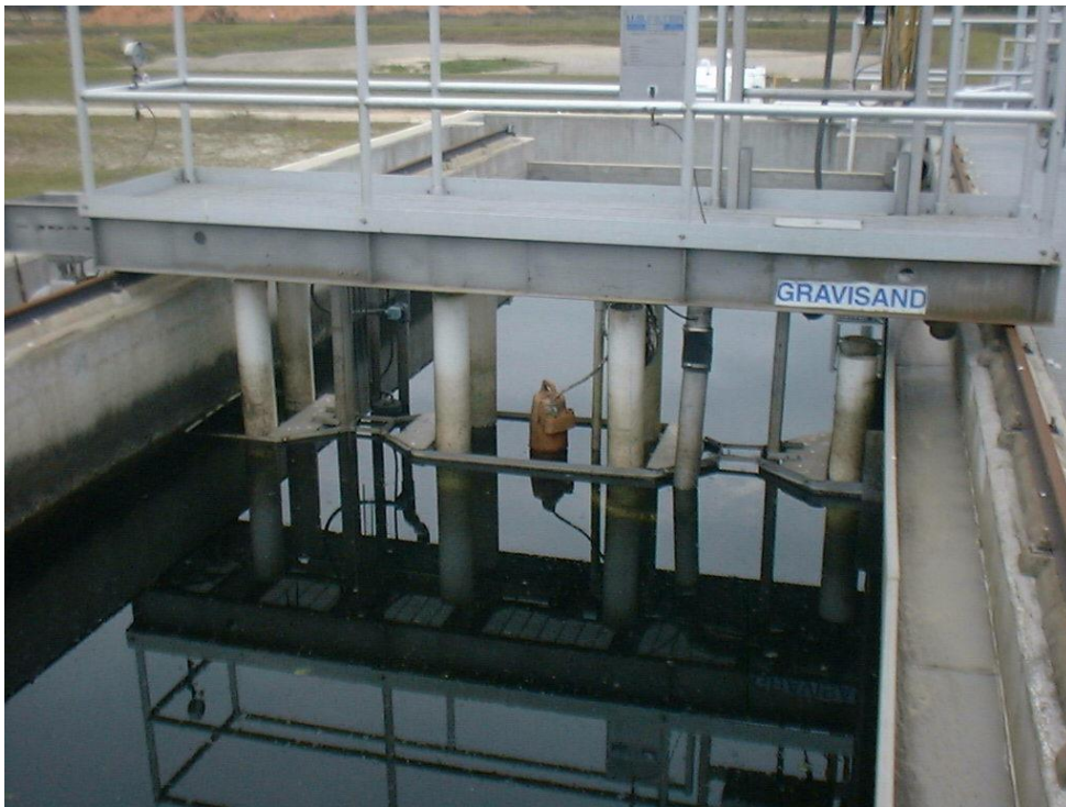
Figure 5.31 - New Traveling Bridge Filter at WWTP5
