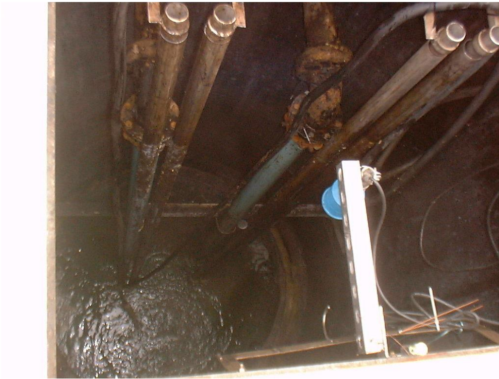
Figure 7.2 – Typical lift station lift station wet well with sonic level indicator
