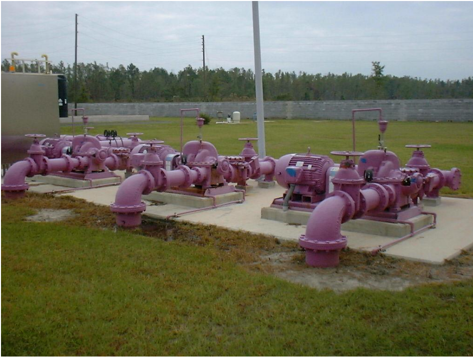
Figure 5.17 – WWTP 2 Reuse pumps
