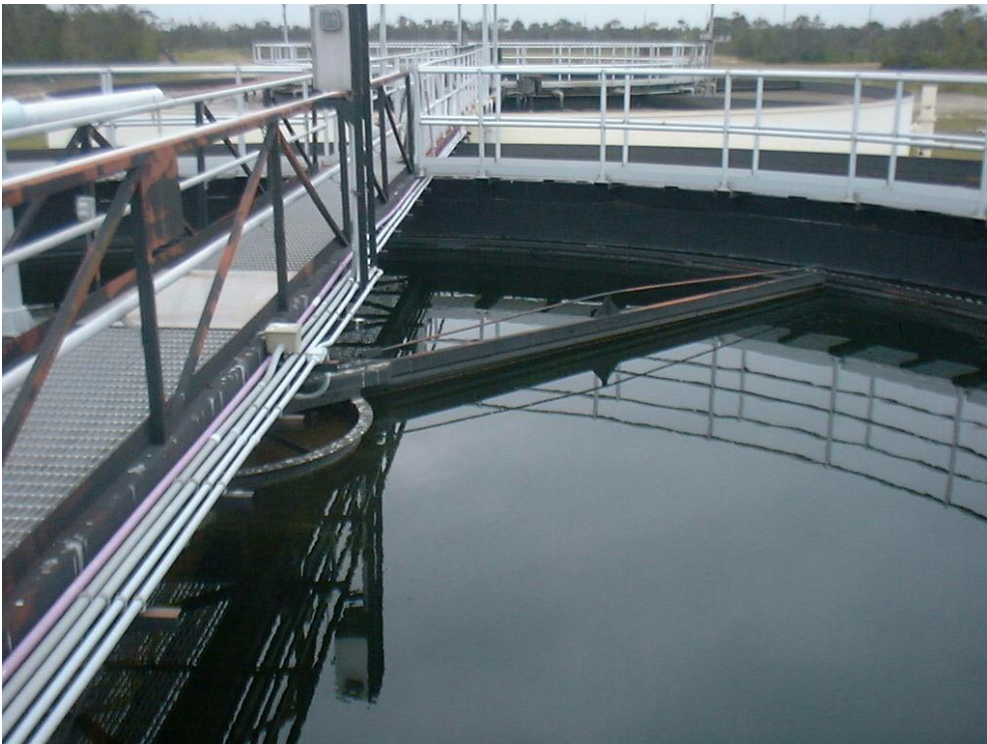
Figure 5.30 - Current aeration basins and center clarifier WWTP 5
