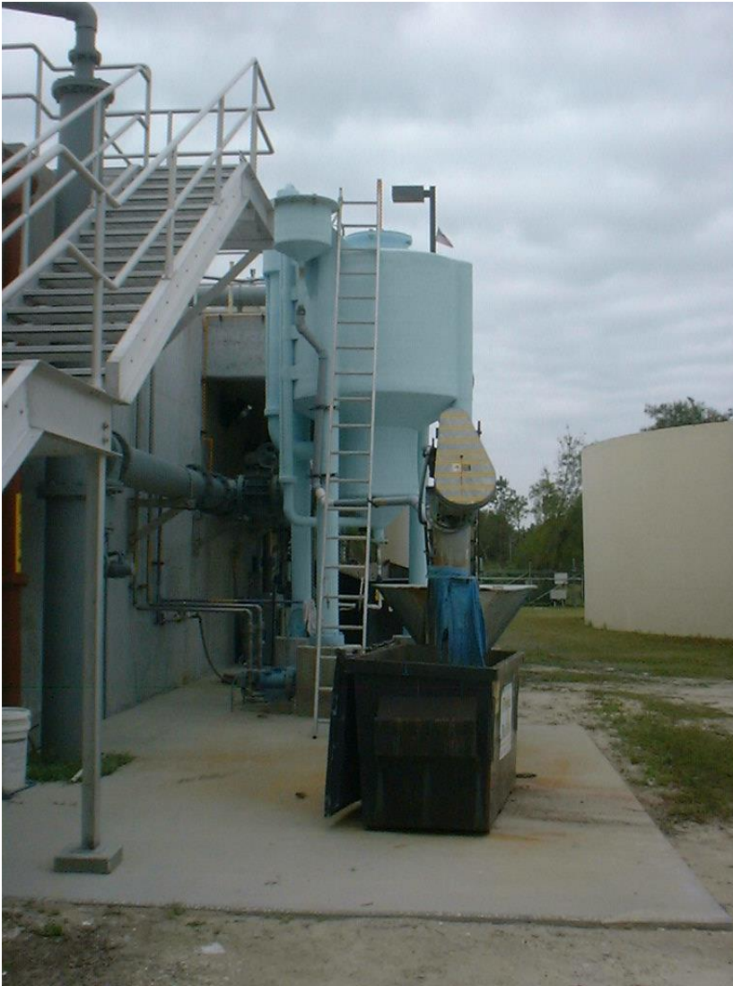
Figure 5.19 – New WWTP 3 influent and grit chamber. The new SBR facility is located beyond the wall on the left. The old package plant, now digester, is seen on the right
