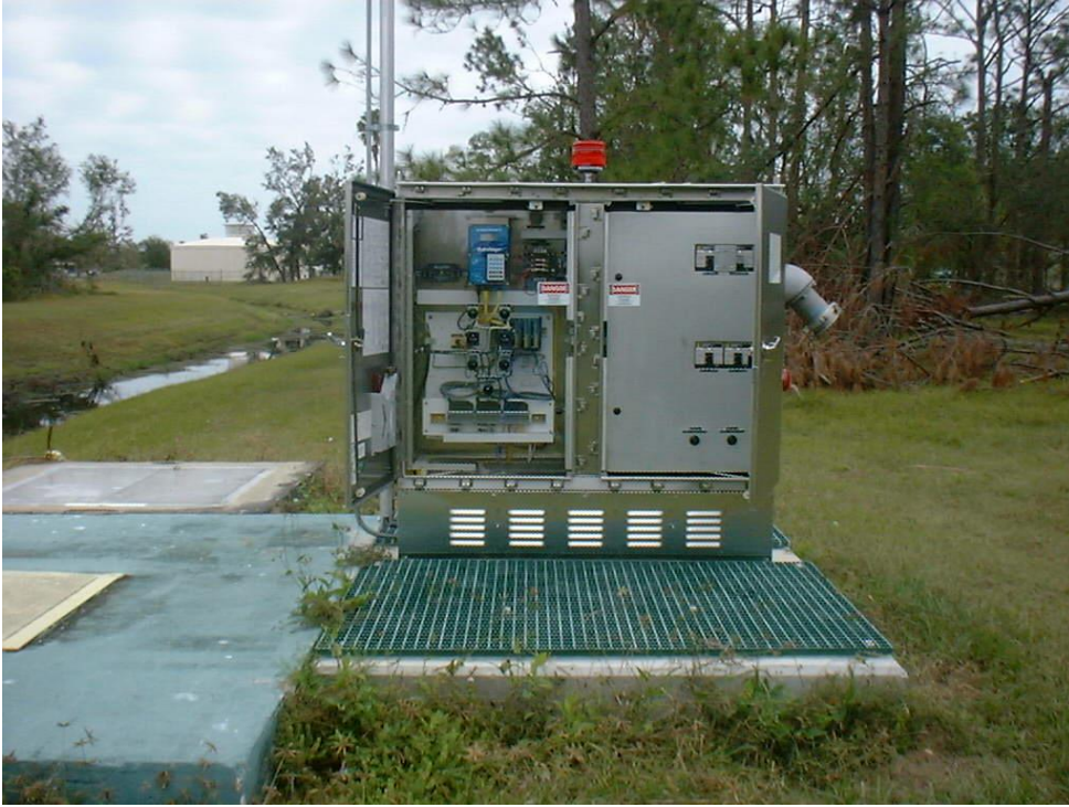
Figure 7.3 - Typical lift station with new standard control box
