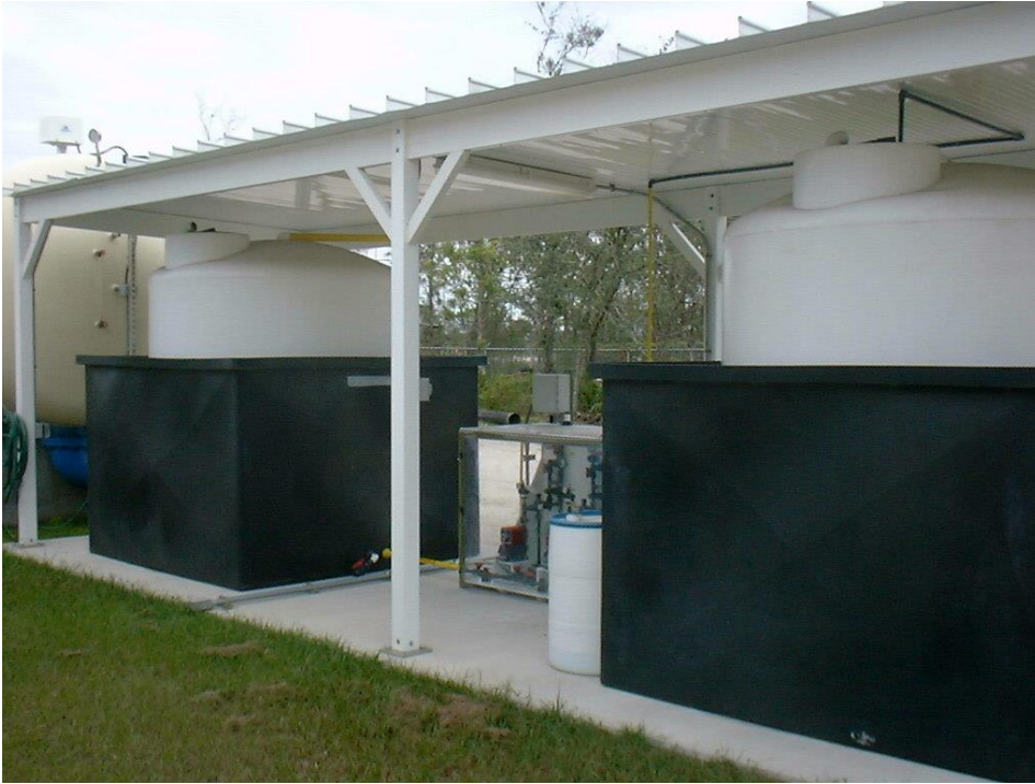
Figure 4.33 - WTP 6 sodium hypochlorite system
