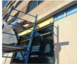
Dens Glass being applied over Hat Channel
