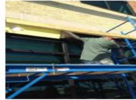
Vapor Barrier being installed over Dens Glass
