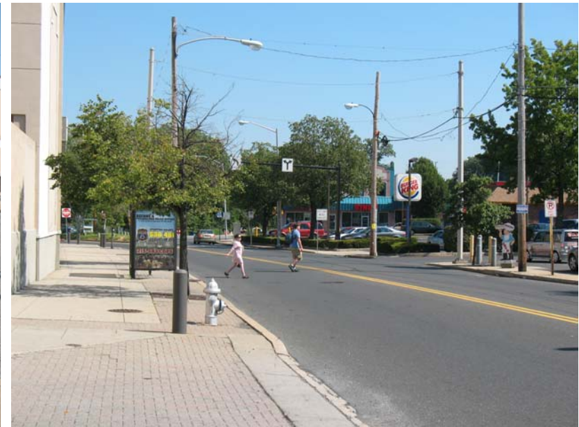
Crosswalks too infrequent for pedestrian-oriented area
