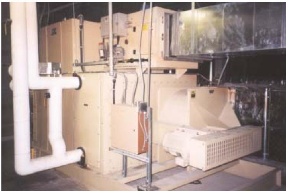
*Drying rooms required dry air entering them to be at 5% RH to maintain a 21% RH room setpoint. Pictured here is a desiccant gas-fired dehumidifier with chilled water post cooling.*
