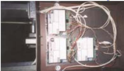
*The clean room control panel: Each zone is controlled through the direct digital control system.*
