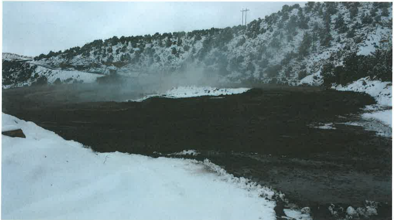
SCA#2 Ash Landfill – working surface looking northwesterly (note steam coming from hot ash with dust control/compaction moisture added)
