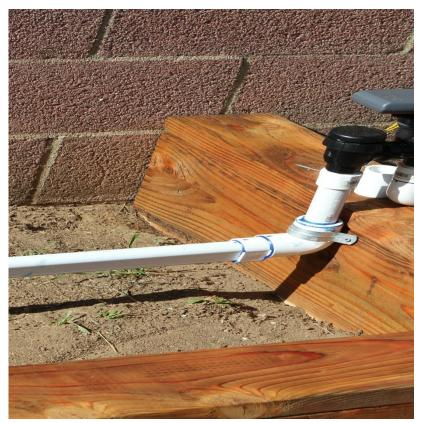
**7.** Mark a line in the center of the PVC el and the top center of the AquaJet this way the AquaJet will be straight up and down and the spray will be parallel with the ground. (See illustration below.)
