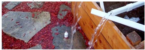
**13.** Glue the round end cap to the Adapter. It now becomes the Adapter/End cap. Glue the adapter/End cap on the end of the system and set it in the trench. Let the glue dry and you are ready to test the system. Turn it on and make sure all the jets are emitting water. After you have tested the system it is now time to cover it up with the soil.
