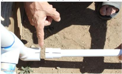
**9.** Now you are ready to glue the second piece of AquaJet into the coupler. Prop the AquaJet up with a board or PVC out of the trench so you do not get any dirt in it while you are gluing onto the AquaJet. First put a thin layer of glue all the way around the AquaJet.
