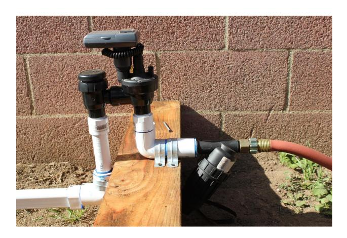
**6.** The bottom of the PVC El should be 3 inches below the surface (soil). The AquaJet Adapter will then be 4 in below the surface because it hangs down lower than the PVC el
