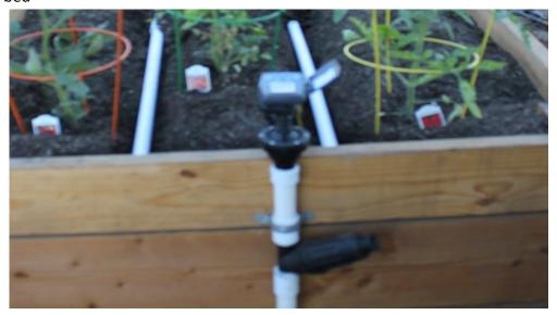
Or install a hose to the filter with the PVC going into the bed. See picture below.
