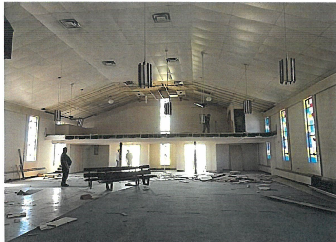
and ended the day with the beginnings of our new facility.
