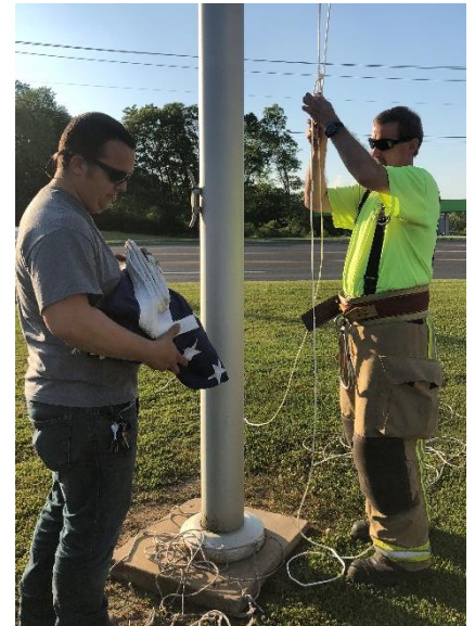
PICTURED ABOVE: CAPTAIN KEVIN CARLISLE RIGHT & FIREFIGHTER TYLER VINCENT LEFT ASSISTED WITH RESTORING A LARGE AMERICAN FLAG AFTER REPAIRS WERE MADE OUTSIDE A BUSINESS AT 1661 AIRPORT ROAD.
