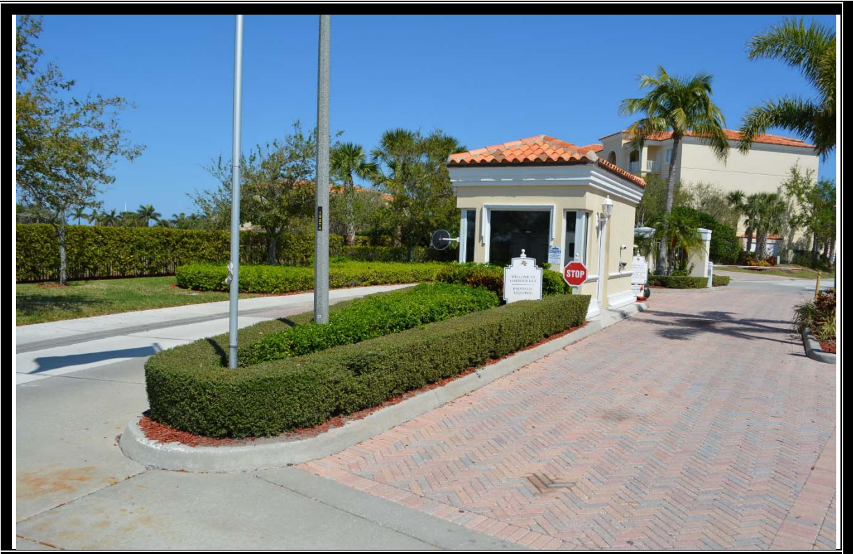
EXTERIOR VIEW OF GUARDHOUSE
