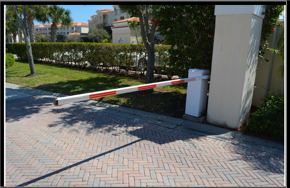
VIEW OF ENTRANCE GATES
