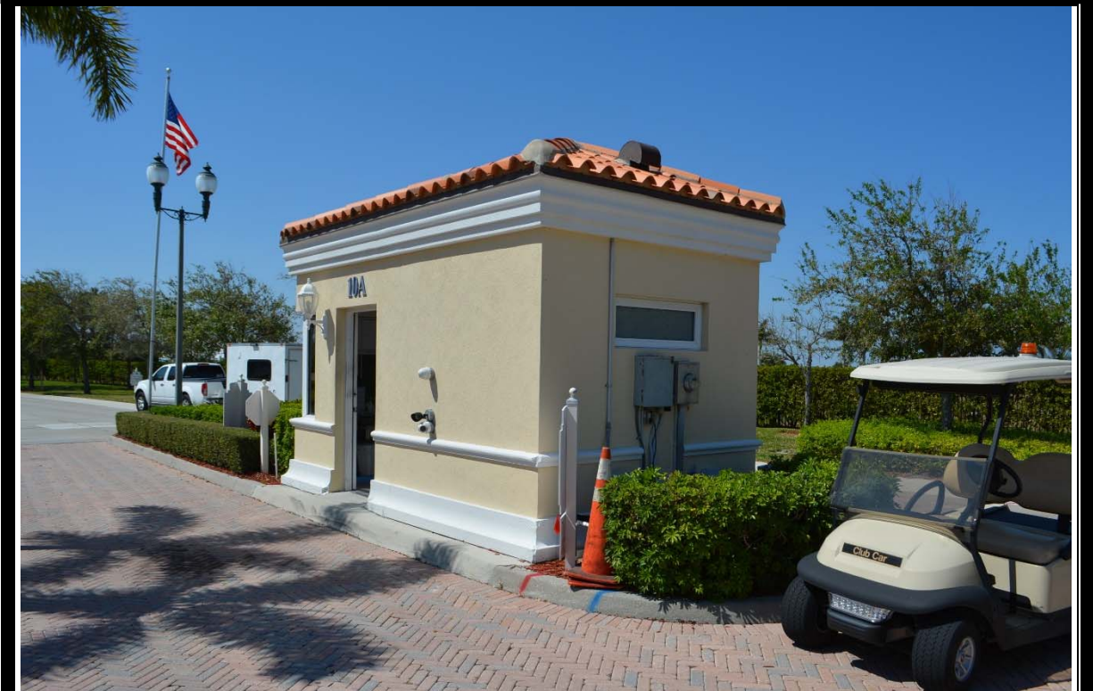
EXTERIOR VIEW OF GUARDHOUSE
