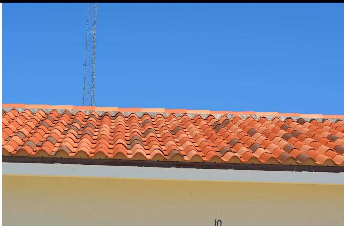
VIEW OF STORAGE/GARAGE BUILDING ROOF
