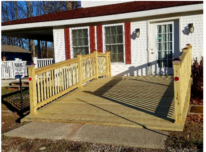
The new access ramp at Haynes House
