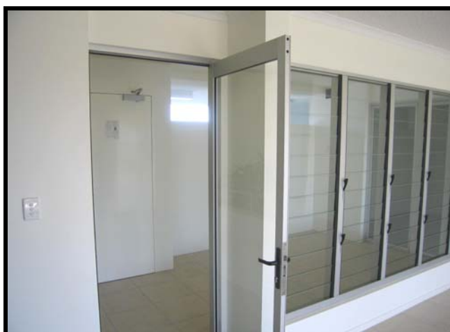
Figure 5 – View from inside unit showing entry door and opening to the “courtyard”. The foreground of this “courtyard” shows lockable windows and door to provide the necessary security
