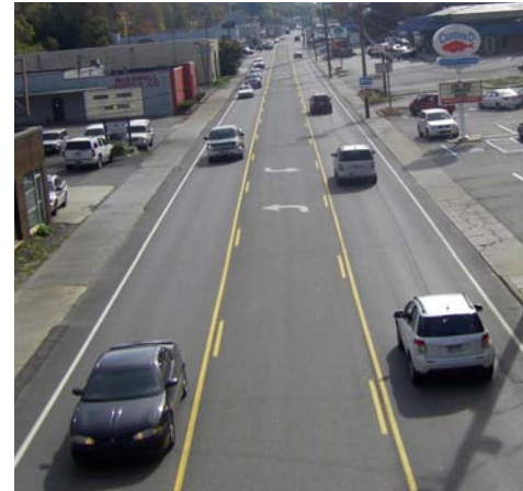
Robert C. Byrd Drive Looking South from Rail Trail Bridge
