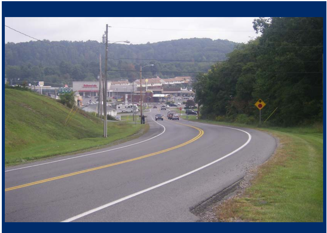
Intersection of Pinewood Drive and Robert C. Byrd Drive Near Area Where New Bypass Will Intersect.
