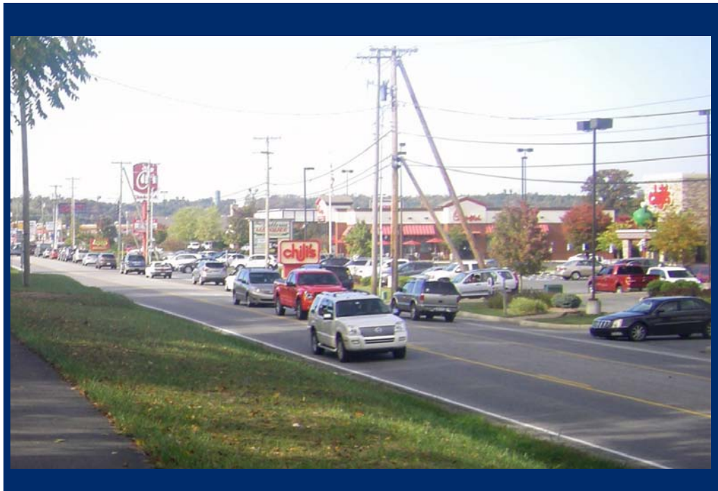
Eisenhower Drive (shown above) is among the City's busiest highways. Traffic volumes north of the area pictured (past the intersection with Robert C. Byrd Drive) exceeded 15,000 vehicles per day according to the most recent State of West Virginia traffic counts.
