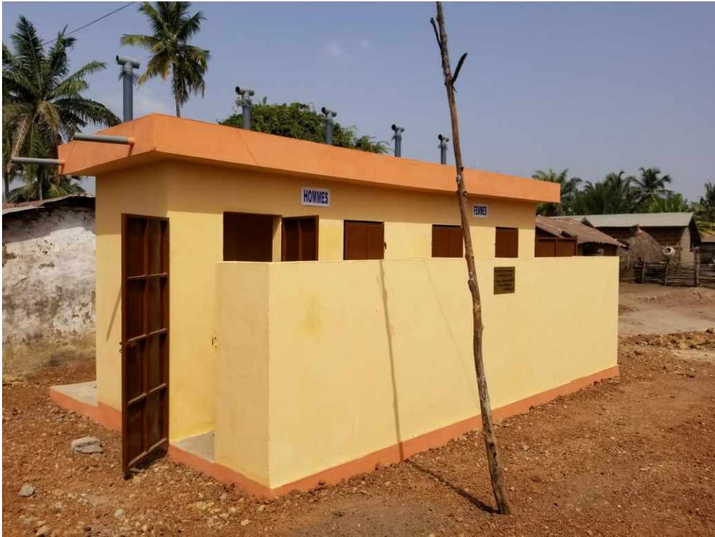
Fig. 31- Side view of completed latrines.
