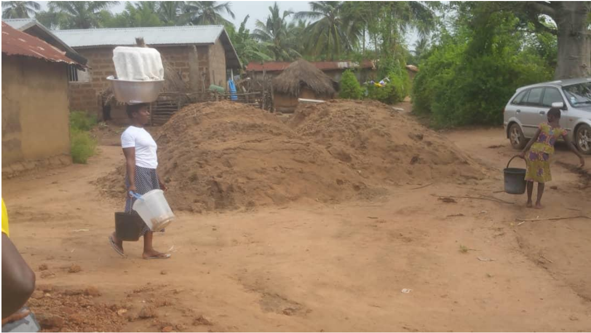
Fig.7- Sand unloaded by truck.
