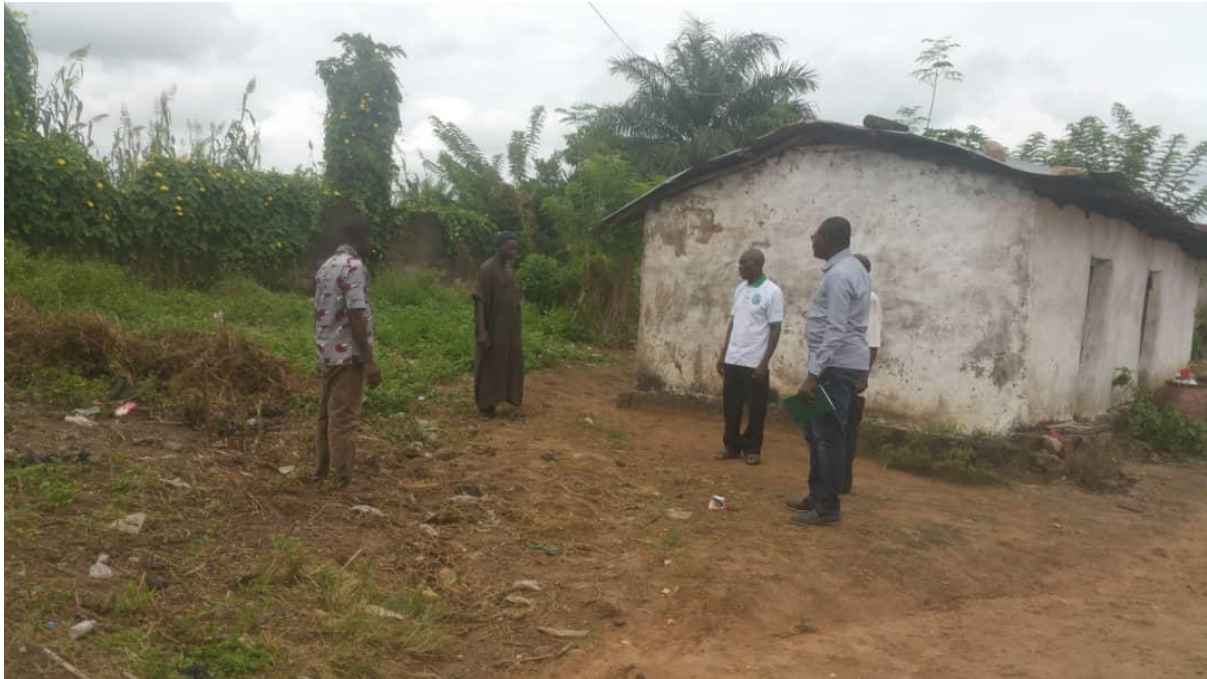
Fig. 6- Beginning of site cleaning.
