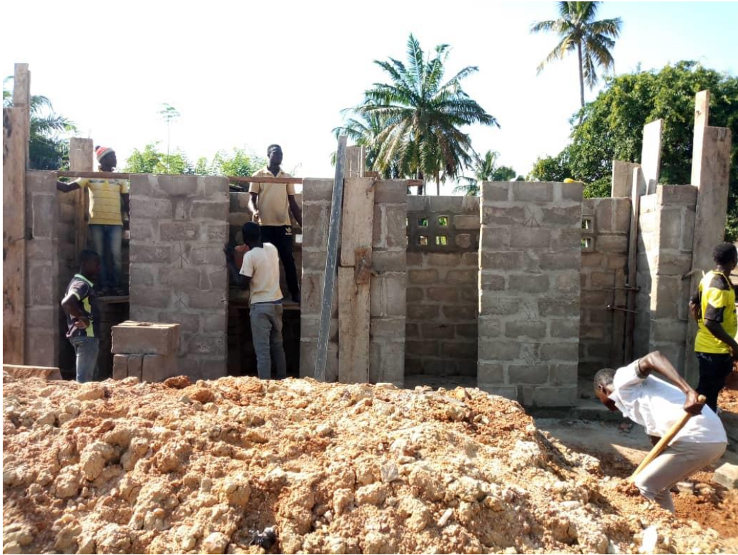
Fig. 14- Cabins walls' elevation.
