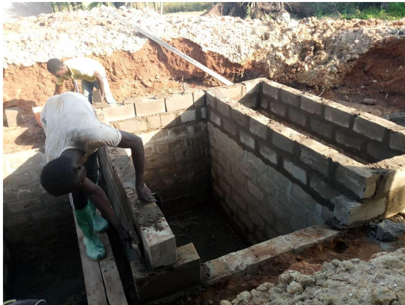
Fig. 12- Septic tank walls building.
