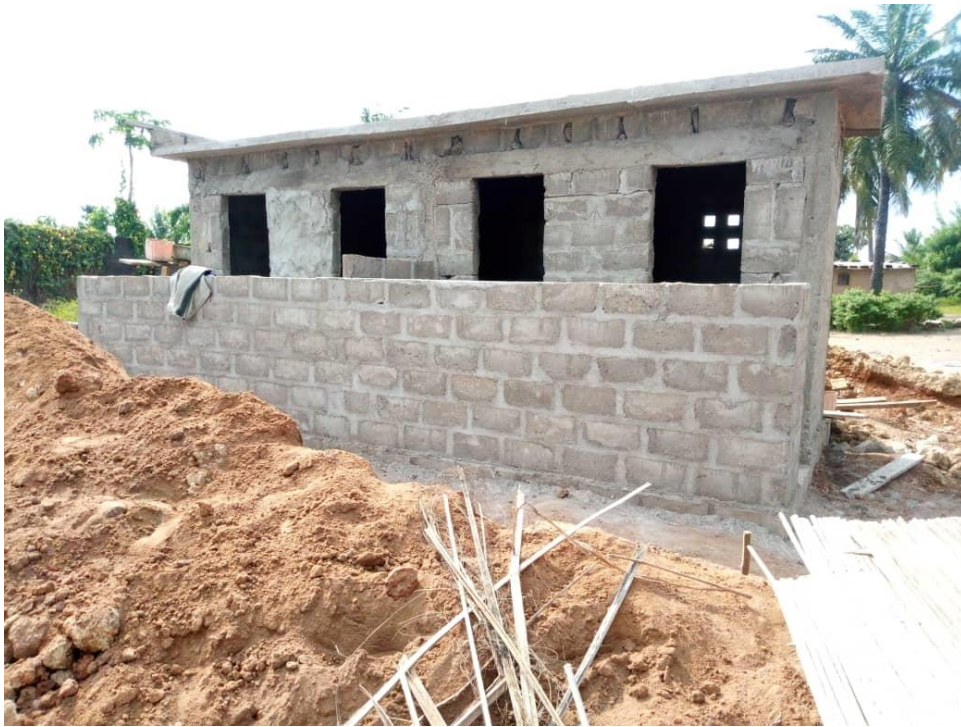
Fig. 15- Cabins walls completed.
