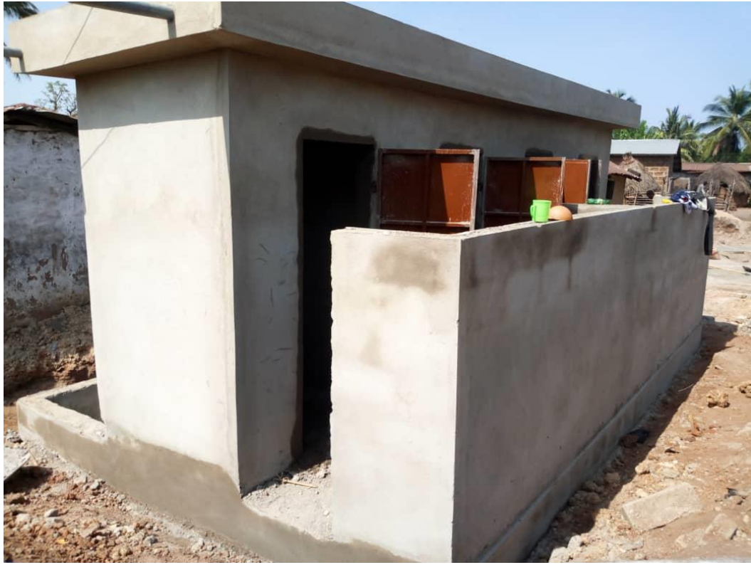
Fig. 18- Plastered cabin walls.
