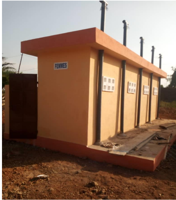
Fig. 23- Latrines back view with closed septic tank
