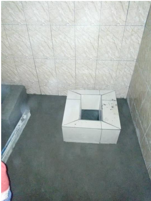
Fig. 21- Interior tiles fixed.
