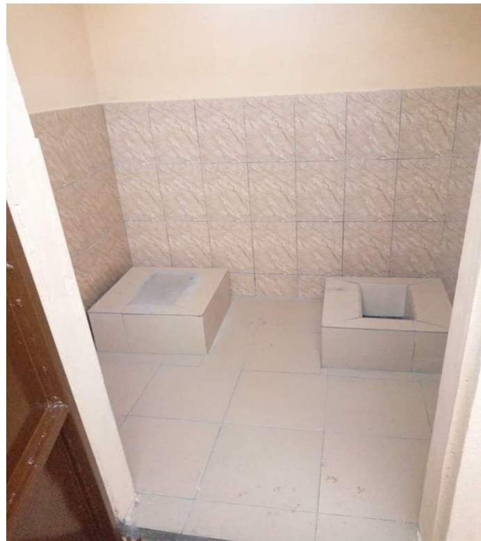
Fig. 30- Inside view of completed latrines
