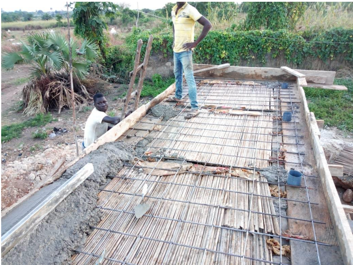
Fig. 13- Laying of cabin's foundation.
