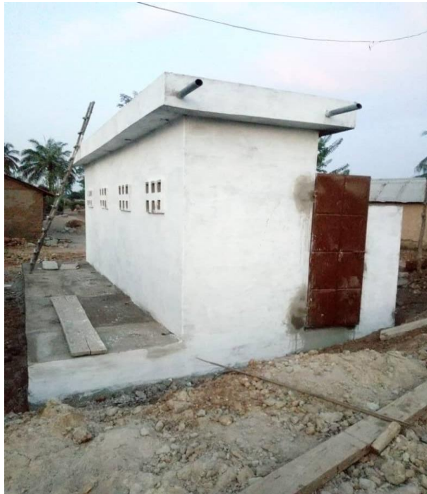
Fig. 22- First paint coating.
