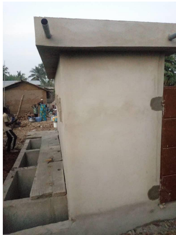
Fig. 19- Back view of cabin plastered walls with septic tank
