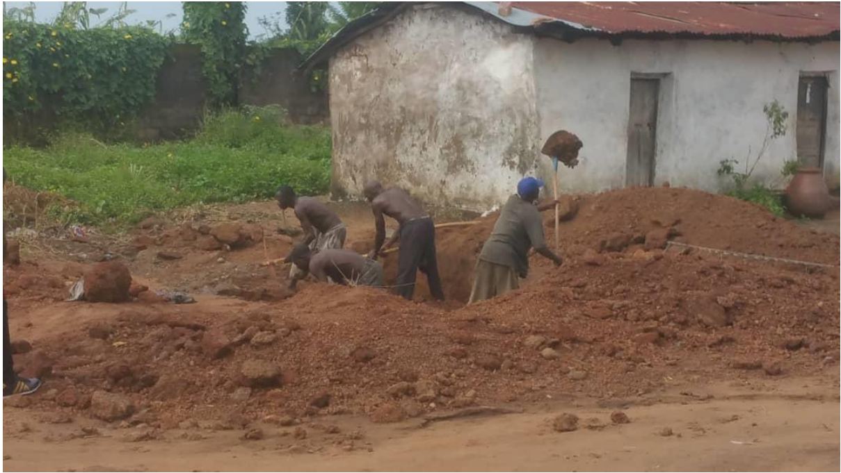
Fig. 11- Digging of the pit for Septic tank.
