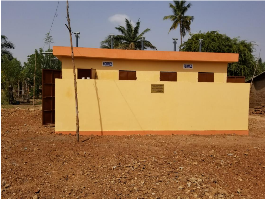
Fig. 29- Outside view of completed latrines.
