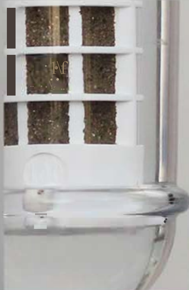
Old Fashioned Spin-Down Filter After Cleaning
