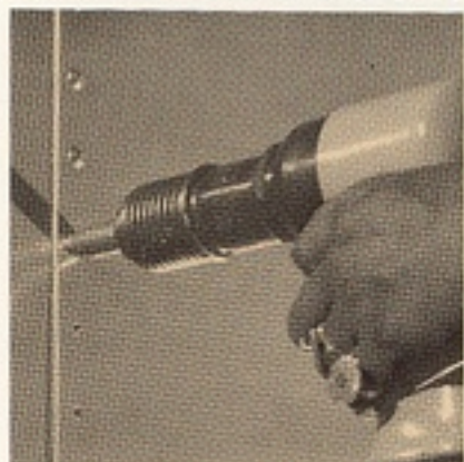
RIVETS BOND EACH SECTION
