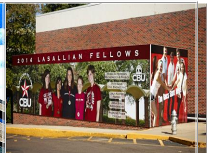
TS44- U-shaped Structure hiding utilities equipment
