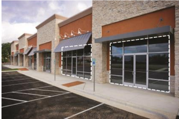
Figure 1220-A: The window area is illustrated within the dashed line area for the two storefronts in the above image.
